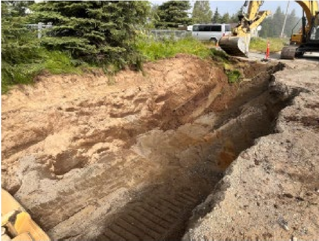
Continued excavation of bury pit near STA 6+85 Repaired sewer service pipes bedded & covered
