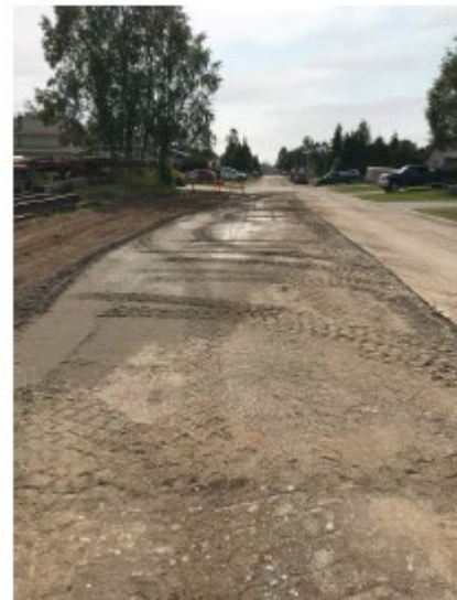
Compacted backfill at Sta 11+14
