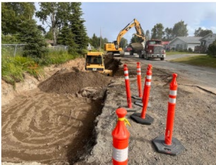
Partial backfill of STA 5+80 to 6+89 excavation
