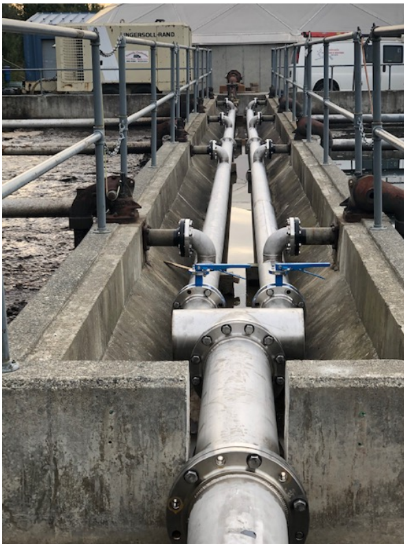
Stainless Piping installed
