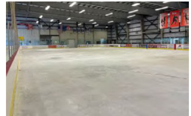
Interior of facility
