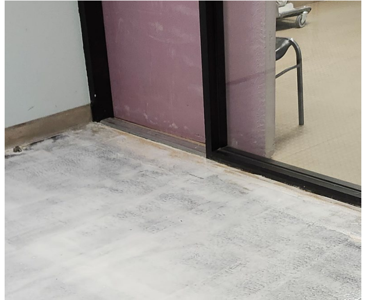
Stripping and priming the floor for the finish
