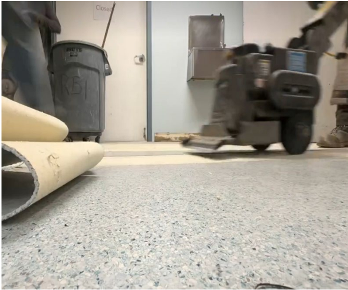
Stripping and priming the floor for the finish
