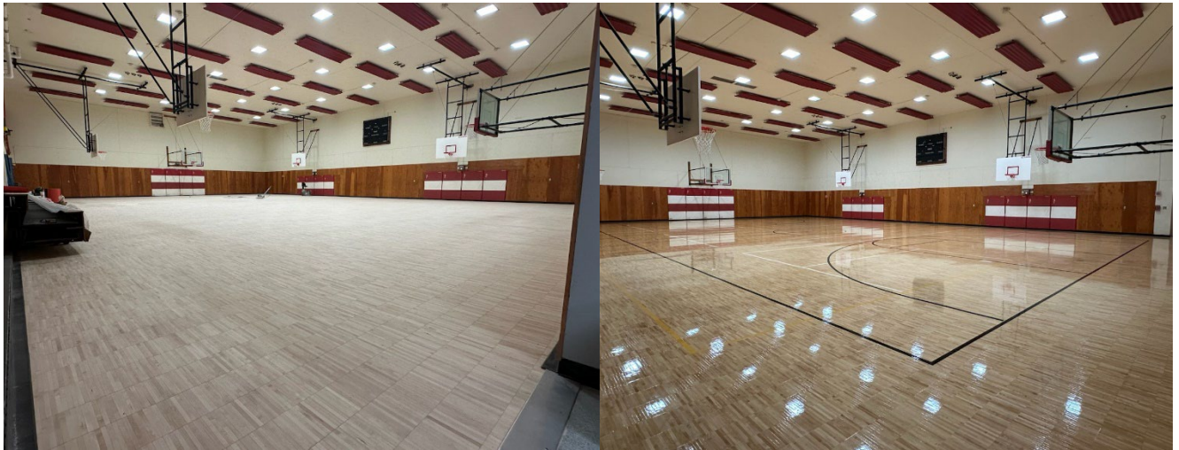
The courts were sanded down and repainted, and 2 coats of finish were put on.
