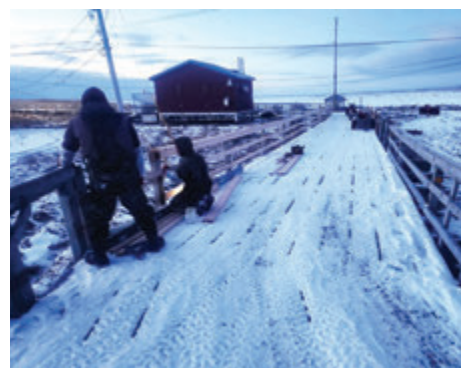
The Knik team replaces critical boardwalk roads throughout the village of Chefornak.
