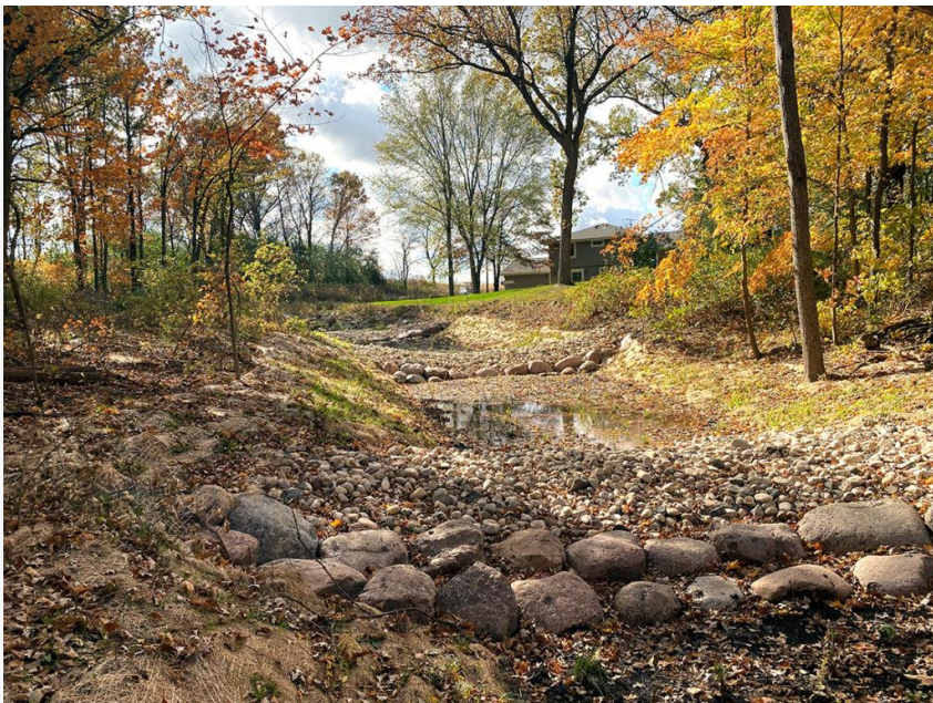
Regenerative stormwater conveyance was effectively used for the Reck South Ravine stabilization project in Kenosha County, WI.
