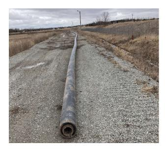
This is the new force main for the leachate collection system. The pipe was fabricated the week of 4/4/22, and expect installation to start the Week of 4/11/22.
