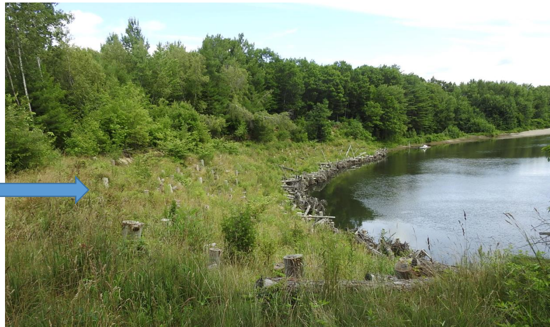
Near stream tree removal replaced with native plantings. Also shows bio-engineering to protect the toe.
