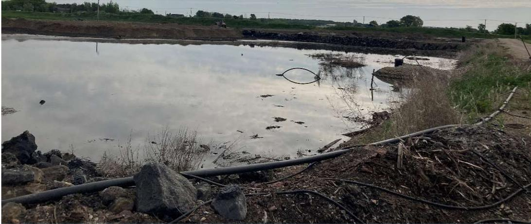
East Module Phase 6 Sequence 1 (This module is nearly full, and surface sump has been rebuilt)
