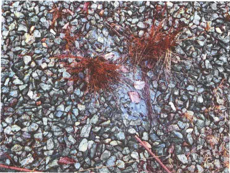
Photo 4 - Course gravel on the surface of the fill pad.
