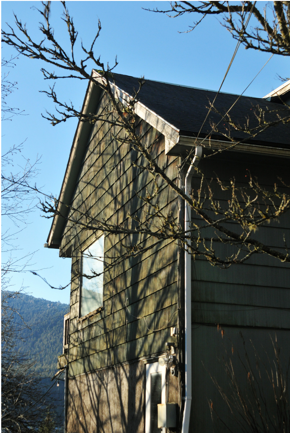
South Facade featuring a contemporary picture window and an entrance to one of the three basement units. Shake-Shingle siding covers the entire residence. Peterson-Kasnick House, 2023
