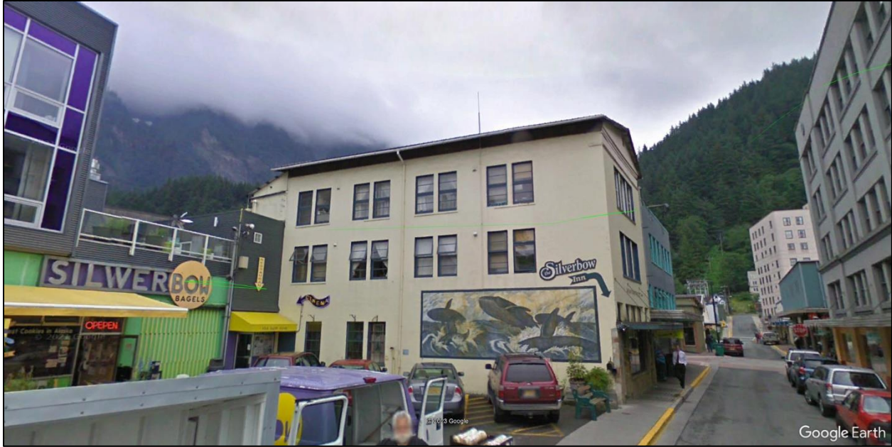
Figure 21. Looking northeast at the San Francisco/Purity Bakery (JUN-00142) from Main St. (photograph courtesy of Google Earth).
