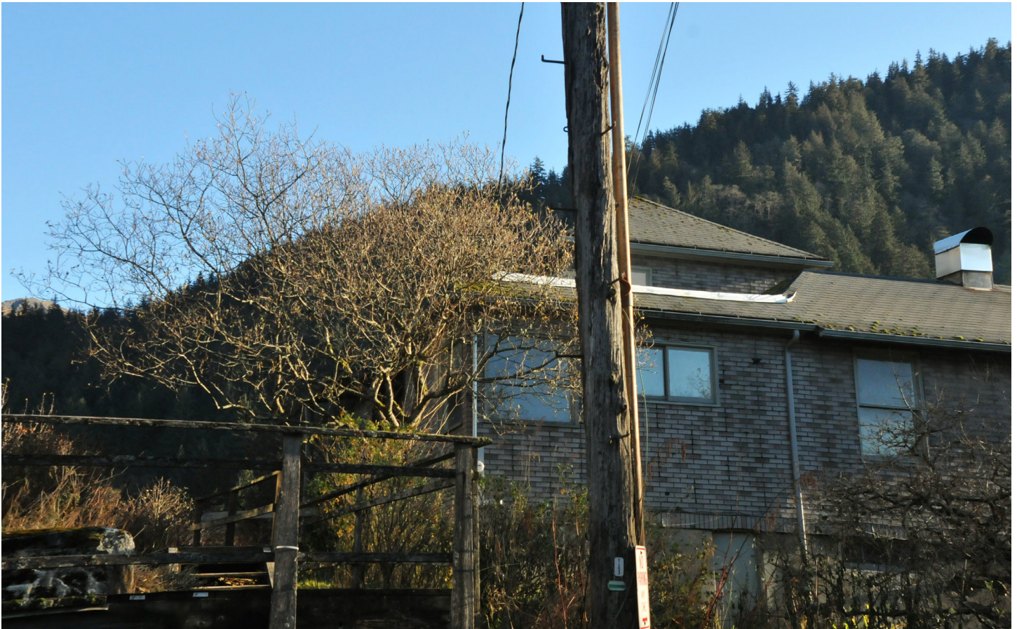
West Facade; Higher roofline reflects the initial, two-story house. Lower roofline shows later renovation encompassing the original house. Edward Webster House, 2023
