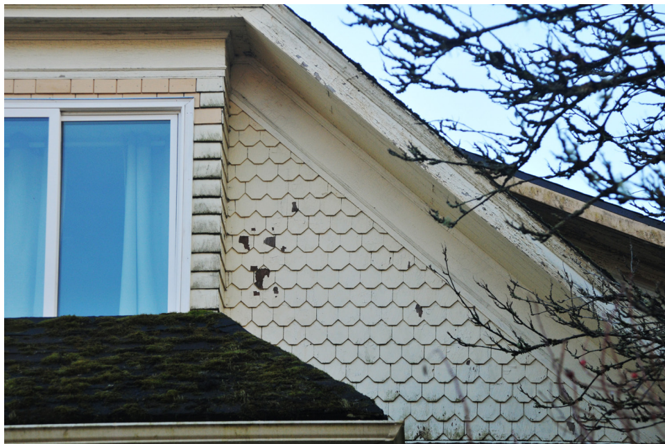
Original scalloped/fish scale siding retained Bosch-Carrigan House, 2023
