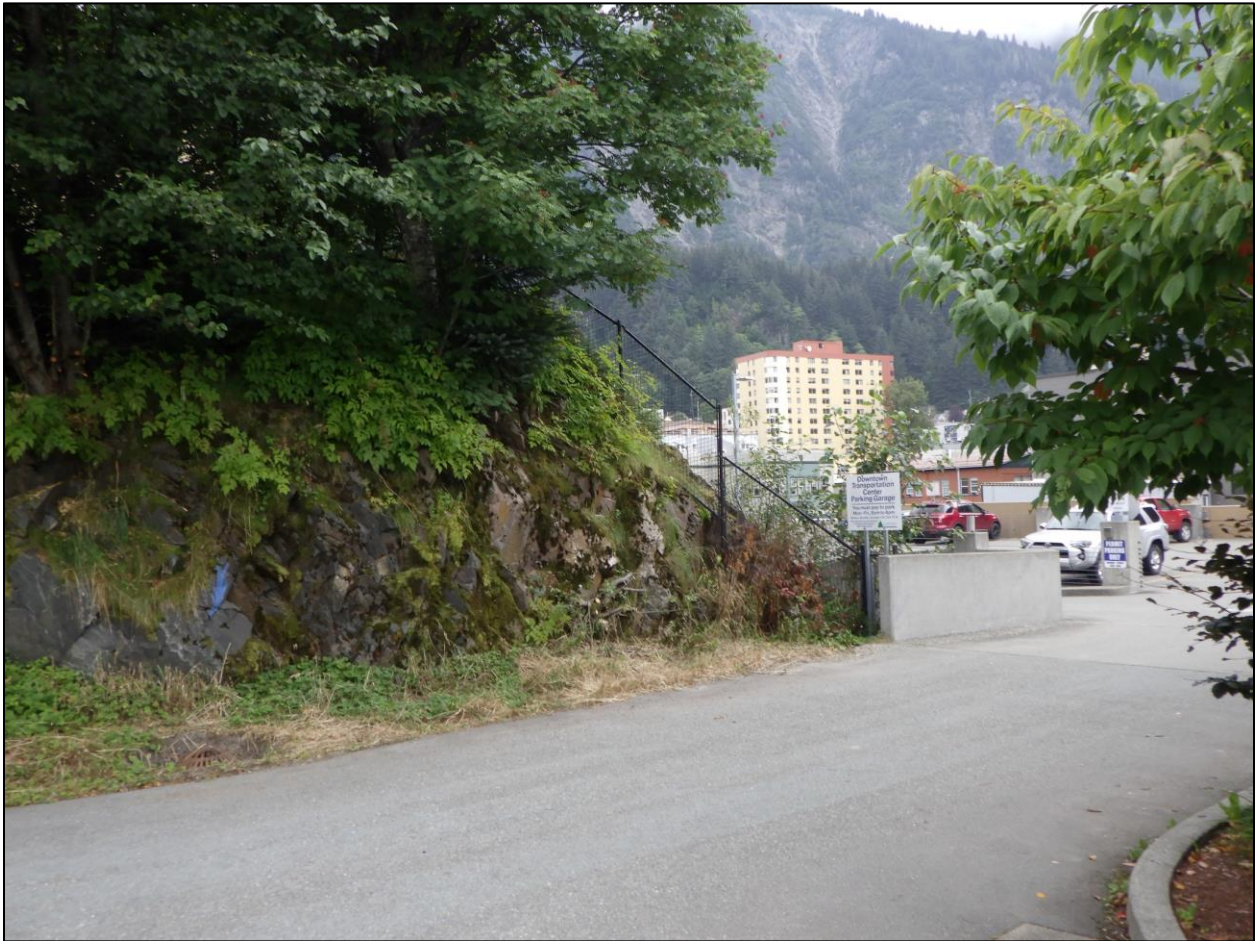
Figure 17. Looking northwest at the former location of the Percy Reynolds House (JUN-00977) showing the site is demolished (NLURA photograph).
