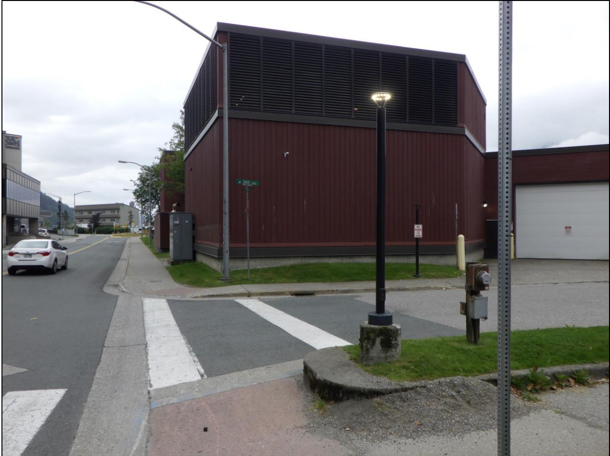
Figure 24. Looking southeast along Willoughby Ave. at the former site of the I.L.W.U. Hall (JUN-00188) (NLURA photograph).
