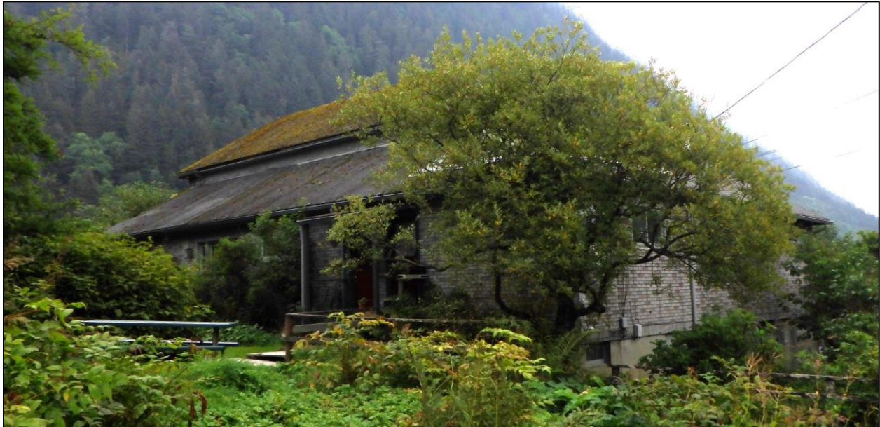
Figure 5. Looking east from Dixon St. at the Edward Webster House (JUN-00070) in 2023 (NLURA Photograph).
