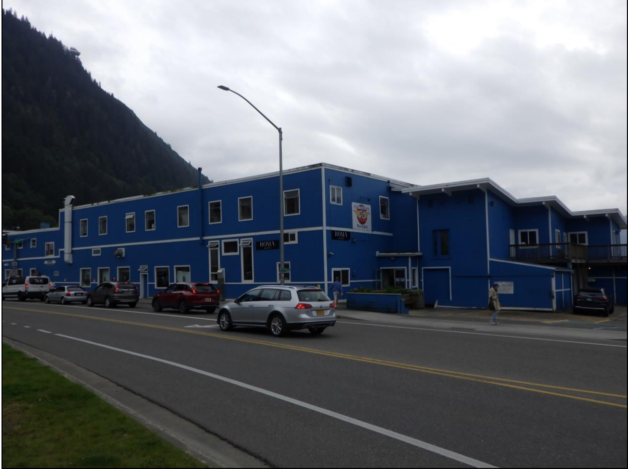
Figure 20. Looking southeast at the Pacific Coastal Steamship Wharf from Egan Ave. (JUN-00120) (NLURA photograph).
