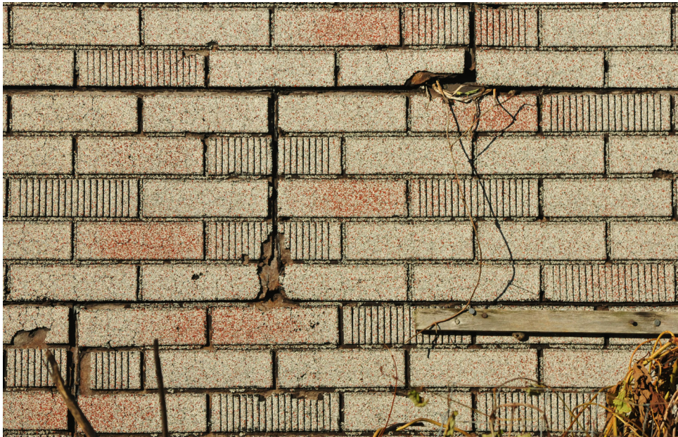
Asphalt-shingle siding covers the original clapboard siding. Therefore the residence does not retain the key exterior materials dating from the period of its historic significance.
