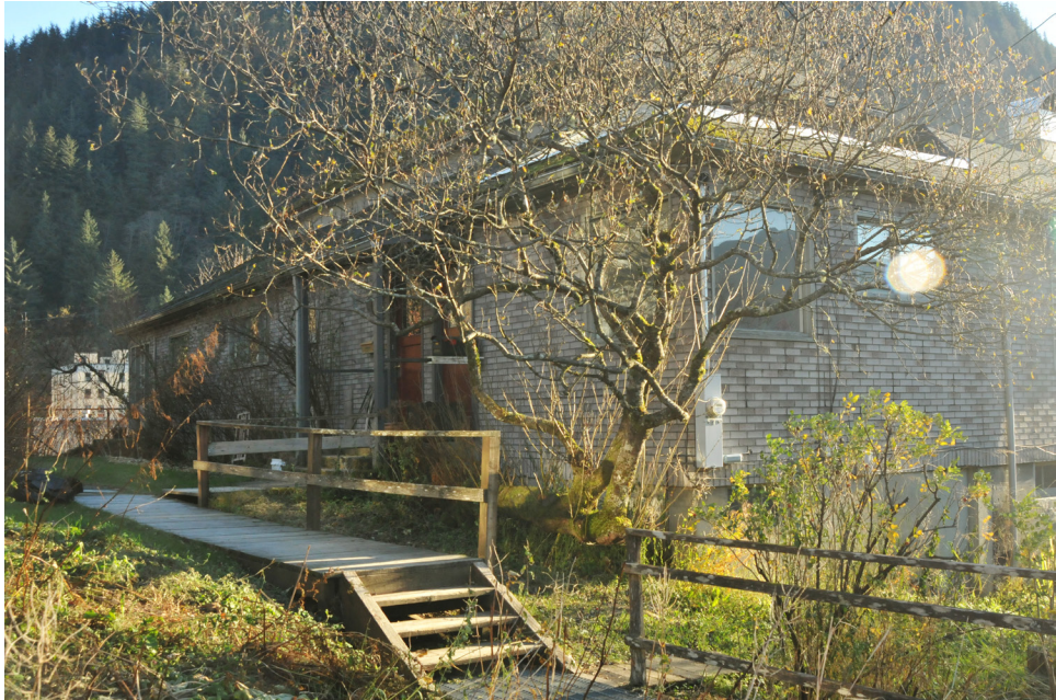
North Facade, main entrance Edward Webster House, 2023
