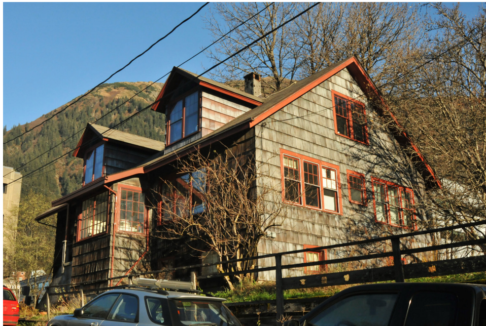
West and South Facades. Bayless-Powers House, 2023
