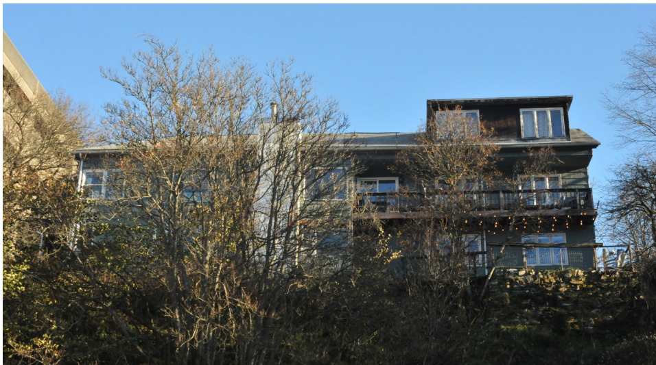
West Facade. Contemporary decks added to allow access to the three basement apartments. The dormer is also a contemporary addition. Peterson-Kasnick House, 2023
