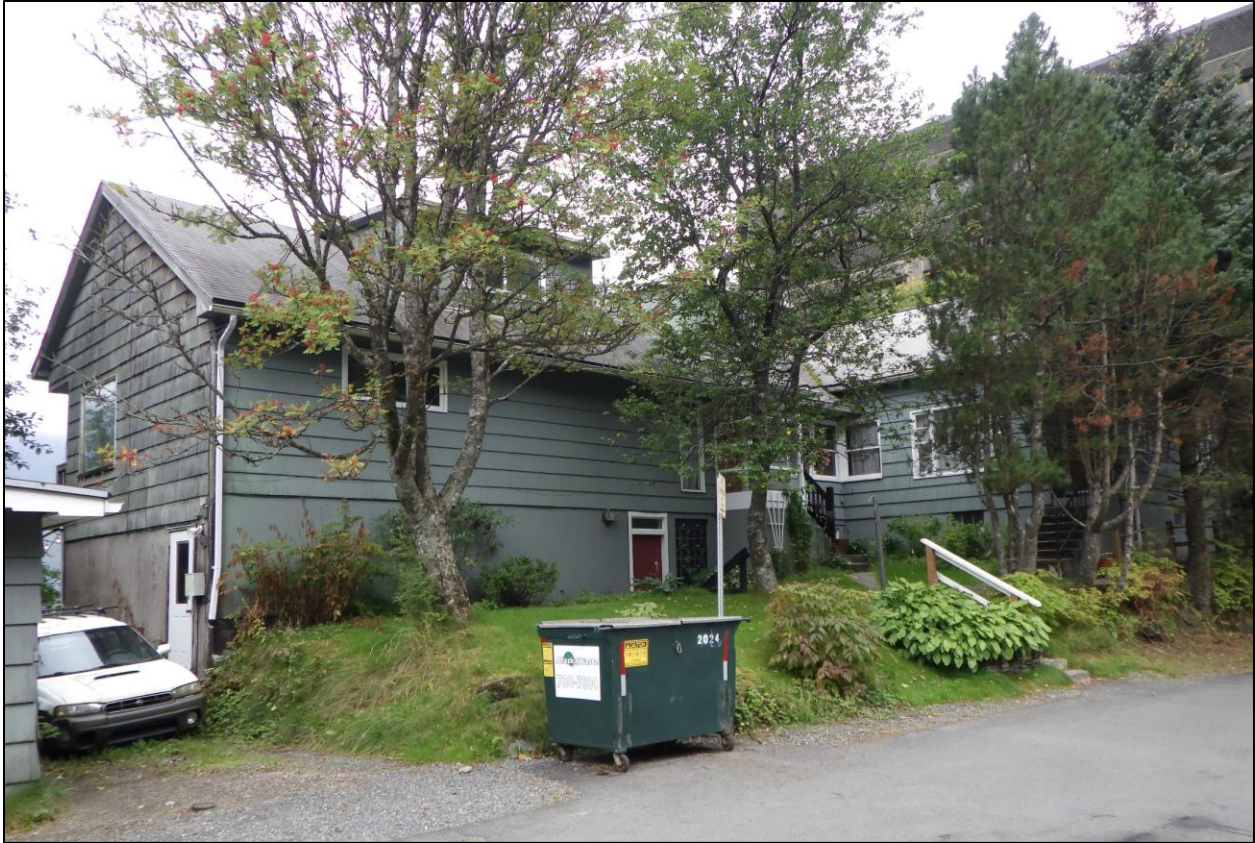
Figure 8. Looking northwest from Dixon St. at the Peterson/Kasnick House (JUN-00292) (NLURA photograph).
