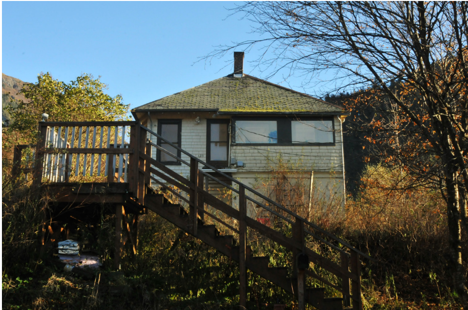
West Facade. Stairs and decks are contemporary additions. Worthen-Hurley House, 2023
