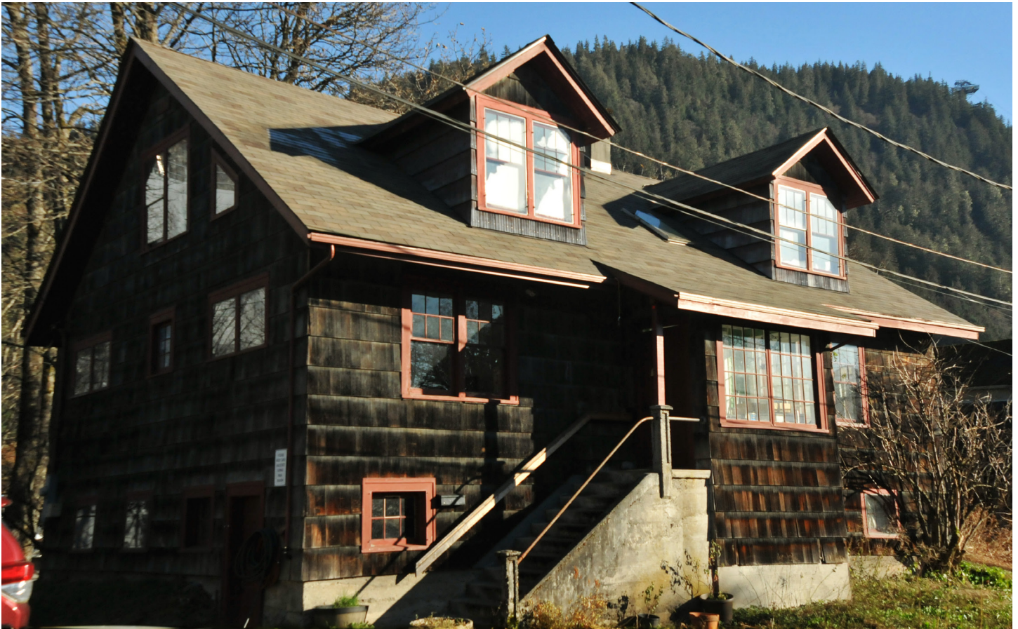
South Facade. Original, double-hung sash windows and original cedar shake siding retained. Wooden gutter has been replicated and replaced in the 1980s. Bayless-Powers House, 2023
