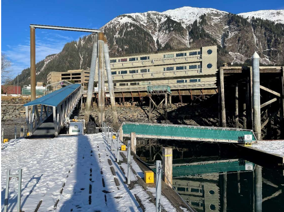
PHOTO 1 – Looking north toward Tidelands CX4 which includes the blue covered gangway and is between the three-story building and the green ramp.
