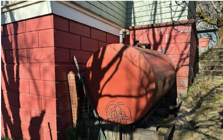
Fig. 19: Storage Tank at 214 Dixon St.
