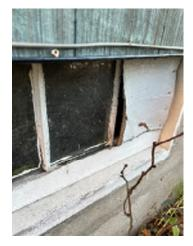
**Figure 7-16.** A Basement Broken Window, Which Is Not Adequately Sealed, That Can Allow Water or Animals Inside.
