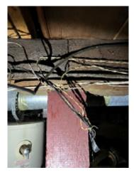
**Figure 7-51.** The Top of the Column Has a Shim. Even if toe-nails were present, it may not reach the beam its supporting.
