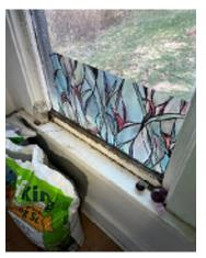
Figure 2-21. Rotting Window Frames.
