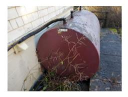
Figure 2-12. Tank Is Not Seismically Anchored.
