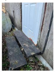
**Figure 7-6.** Unprotected Plywood Sheathing by the Siding and Rust Around the Man Door.
