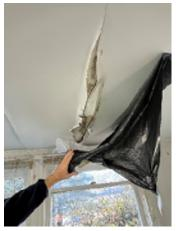
Figure 3-32. More Damage From a Roof Leak Under the Bag.
