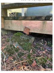
Figure 7-23. A Rotated Walkway Support Connector.
