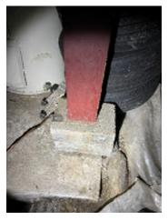
**Figure 7-50.** The Column Is on a Concrete Block That Is Not Sitting Fully on the Concrete Below.
