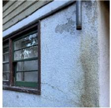
Figure 1-6. The Drainpipe Ends Abruptly in Mid-Air and Does Not Direct Water Away From the Foundation.
