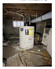
Figure 7-53. The Tank Is Not Seismically Secured.
