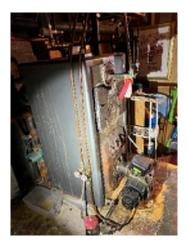
**Figure 2-33.** Signs of Leaks Exist With the Staining on the Side of the Unit.
