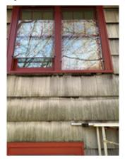
**Figure 6-9.** Deteriorating Window Sill.
