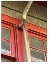
Figure 6-11. Drainpipe Is Rusted.
