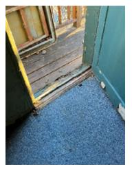
**Figure 2-32.** Door Jam Is Rotten. The door does not fully seal in the frame.
