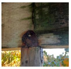
**Figure 1-3.** Rusted Hardware Connections on the Deck Framing.
