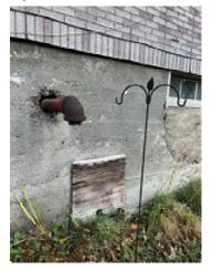
**Figure 4-10.** Large Hole Where Pipe Exits the Basement and Cracking Between the Different Concrete Pours Under Window.
