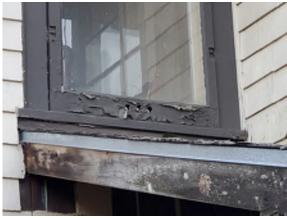
**Figure 2-2.** Three Holes in the Window That Could Allow Water to Enter the Building.
