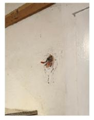
**Figure 3-28.** Exposed Wiring Was Observed in Multiple Locations, Creating a Hazard. One location did not have wires caps.
