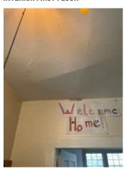
Figure 6-20. Cracked Drywall and Drooping Ceiling.
