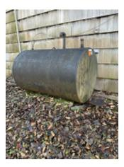
Figure 6-8. Fuel Tank Is Not Seismically Anchored.
