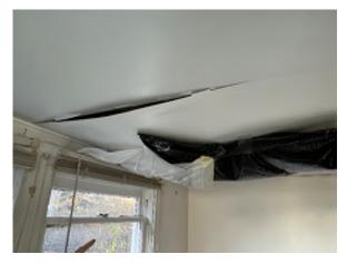
**Figure 3-31.** Ceiling Damage From a Roof Leak.
