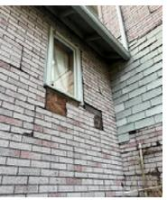
**Figure 4-8.** Deteriorated/Missing Siding.
