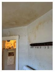
**Figure 3-25.** A Significant Amount of Discoloration on the Sheetrock Above the Stove in the Kitchen, Water Damage.
