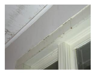
Figure 5-26. Indications of Water Damage on Windowsill.
