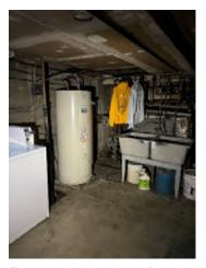
Figure 7-46. Water Heater Does Not Have Seismic Straps.
