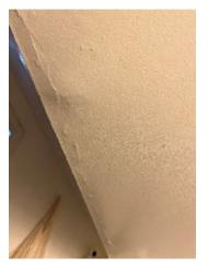
**Figure 7-37.** Paint Is Chipped, and the Sheetrock Fasteners Are Visible in Some Places.
