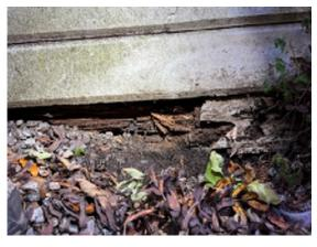
**Figure 1-16.** Exposed Wood Beneath the Siding Is Rotten.
