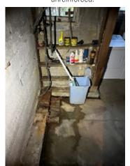
**Figure 7-47.** Multiple Signs of Water on the Basement Floor. There is a small trench for water around the perimeter.
