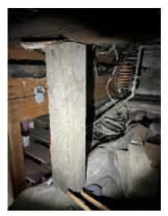
**Figure 7-48.** One Column Is Sitting on the Bedrock With No Connections. There are shims at the top of the column.
