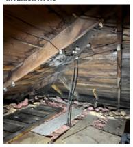
**Figure 4-13.** Cut Rafter Member and Extensive Water Damage From Past Events.
