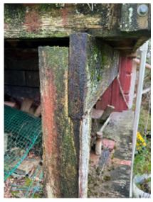
Figure 5-12. Rotten Beam Support and Deck.
