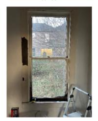
Figure 2-22. Rot in the Window Frames.
