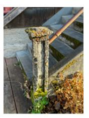
Figure 6-3. Damaged Concrete Post.
