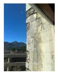
Figure 7-14. Concrete Falling Off the Side of the Chimney.
