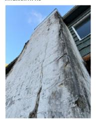
Figure 7-13. A Long Crack Up the Side of the Chimney.
