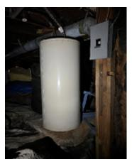
**Figure 7-52.** The Tank Is Not Seismically Secured.
