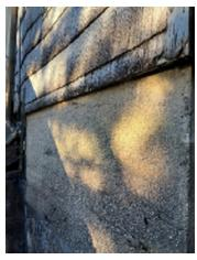
Figure 3-17. Long Crack at the Top of the Wall.
