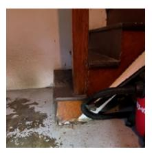
**Figure 1-29.** Wood at the Bottom of the Stairs Has Some Water Damage.
