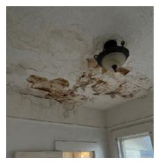
Figure 2-17. Significant Water Damage to the Ceiling
