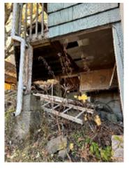
**Figure 7-18.** Missing Soffit Panels. The column is sitting on a concrete pile.
