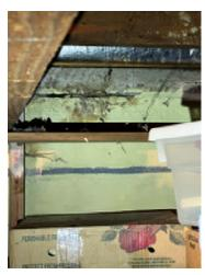
**Figure 5-32.** Large Crack on the Interior of the Concrete Basement Wall.
