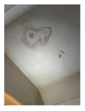
**Figure 2-23.** Water Damage, Cracks, and Exposed Wiring in the Closet on the Northeast Side of the Building.
