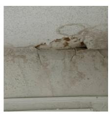
Figure 2-18. Ceiling Paint Is Cracked and Falling From the Water Infiltration. How extensive the water damage is or if there is mold is unknown without a destructive investigation.
