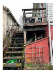
**Figure 5-10.** Rotted Deck and Stairs. Deck posts are not anchored and have no positive connection to joists.
