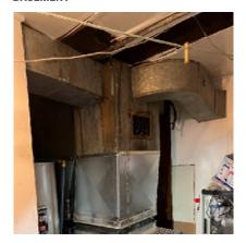
Figure 1-25. Staining on the Ducting Indicating Past Leaks.
