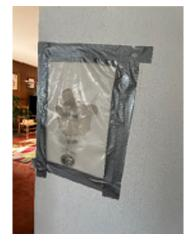
**Figure 7-34.** Mold Is Growing Under the Vapor Barrier. The Extent of Damage in the Wall Cavity Is Unknown.
