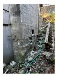
**Figure 3-15.** Failed Chimney Foundation Wall. Collapse Hazard.
