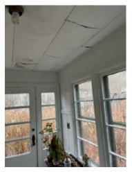
**Figure 4-21.** Sagging Ceiling and Signs of Water Damage in the East Entryway.
