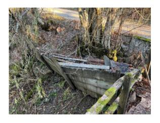
Figure 3-8. Failed Wooden Retaining Wall.
