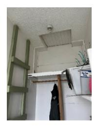
**Figure 2-19.** Inadequate Framing to Support the Closet Used for Attic Access.
