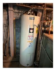
Figure 3-40. No Seismic Strapping Around the Water Heater.
