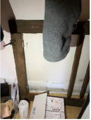
**Figure 3-36.** Sheetrock Crack in the Closet and Mold on the Baseboard.
