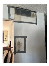
Figure 7-33. Damage to the Finishes Caused by the Sink Leak.
