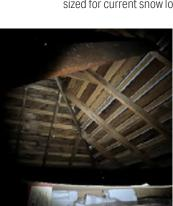
Figure 2-15. Daylight Is Visible Through Holes in the
