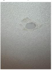
Figure 5-27. Water Damage Around Light Wiring Cover.
