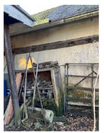
**Figure 5-17.** Gutter Drainage Splashed on the Garage and Caused Significant Moss to Grow and the Plywood to Rot.
