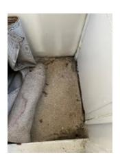
**Figure 7-30.** Moisture Damage and Rot in the Back Entryway.
