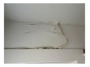
**Figure 4-24.** Cracked and Bubbled Paint likely from Water Infiltration.
