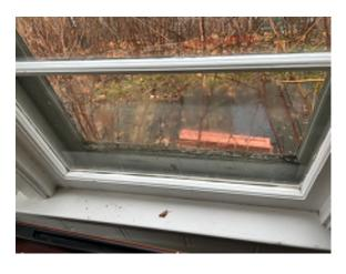
$\textbf{Figure 4-22.} \ \ \, \textbf{Rotting Storm Window and Window Frame}.$
