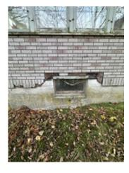
Figure 4-6. Deteriorated Siding and Windowsills.
