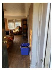
**Figure 3-19.** The Floor Slopes Downward Toward the East Wall and the Door Rubs on the Floor.
