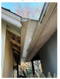
Figure 5-18. Deterioration Under the Eave.
