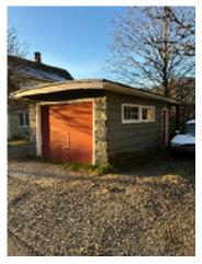
**Figure 7-25.** Garage/Shed on the South Side of the Building. No Lateral System on Front.
