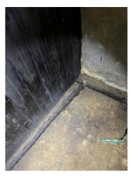
Figure 4-33. Trench Around the Perimeter for Water Flow.
