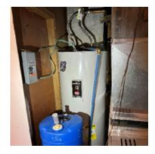
Figure 1-26. Water Heater Without Seismic Strapping.
