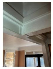
**Figure 3-30.** A Beam Hanger Observed at the Framing Near the Stair Opening.
