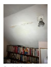
**Figure 6-18.** Cracking and Indications of Water Damage on the Ceiling.
