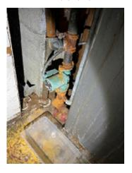
Figure 2-34. Signs of Leaks Exist at the Pipe Connections.
