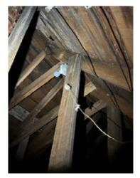
Figure 5-19. Indications of Water Damage on the Roof Rafters.
