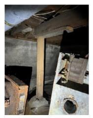
Figure 7-49. A Large Shim at the Top of the Column.
