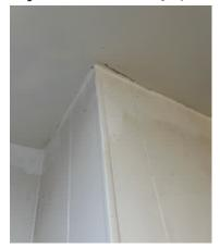
Figure 5-24. Continuous Ceiling Crack Around a Corner.
