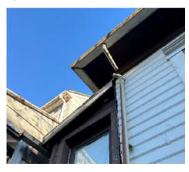
**Figure 1-10.** The Drainpipes Are Disconnected, and Water Is Not Directed Away From the Building.
