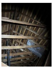
Figure 2-13. Attic Trusses and Most of the Wood Appears Dry.
