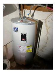
**Figure 2-36.** No Seismic Strapping Around the Water Heater.
