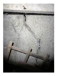
**Figure 1-13.** Visible Wood Framing in the Deep Crack Where Water Infiltrates the Basement.
