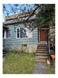
Figure 7-3. Moss on the Concrete Stairs.
