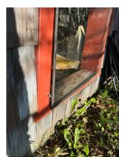
Figure 6-13. Gap in the Storm Window.
