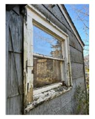
**Figure 3-10.** Rotten Windowsill and Siding in Poor Condition.
