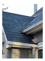
Figure 3-3. Plant Growth indicates Build-up in Gutter.
