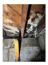
Figure 4-32. Rotting Floorboards.
