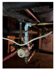
**Figure 2-35.** Signs of Leaks and Corrosion Exist at the Pipe Connections.
