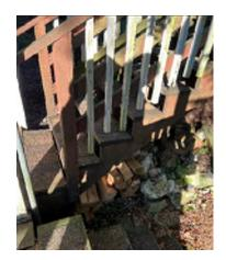
Figure 1-20. A Long Crack on the Side of the Stringer.
