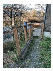
Figure 7-8. Leaning Handrails.
