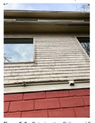
**Figure 5-6.** Deteriorating Siding and Eave.
