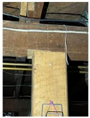
**Figure 5-29.** Shimmed Column With No Positive Connection to the Beam.
