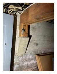
Figure 4-34. Nonstandard Beam Support.
