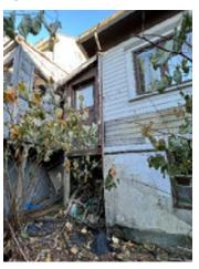
**Figure 1-9.** A Door More Than 6 Feet Above Ground With No Stairs.
