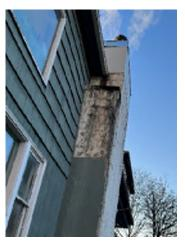
Figure 7-15. Water-Stained Chimney With Visible Cracks.
