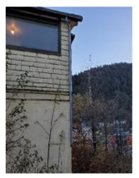
**Figure 2-4.** Drainage Pipe Ends Abruptly Mid-Air and Not Directing Water Away From the Foundation.
