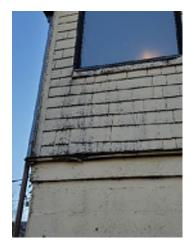
**Figure 2-7.** Black Mold on the Siding at the Southwest Corner.
