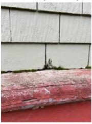
**Figure 5-4.** Deteriorated Siding With Moss Growing in the Gaps.
