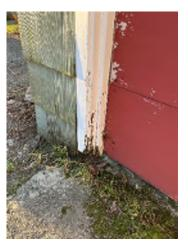
Figure 7-26. Rot Near the Ground.
