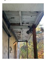
**Figure 3-9.** Peeling Paint and Fixtures Missing Bulbs; Open Fixtures or Exposed Wiring Can Be Hazardous.
