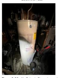
**Figure 6-26.** No Seismic Strapping on the Water Heater.
