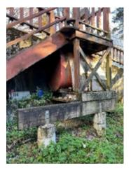
**Figure 1-17.** Fuel Tank Wedged in the Space Under the stairs.
