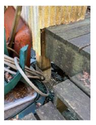
**Figure 7-19.** Moss Growing on the Deck. The column is shimmed and sitting on a concrete pile.
