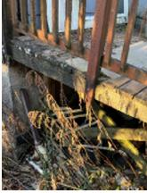
**Figure 3-2.** Drainpipe Is Disconnected and the Deck Framing Appears Rotten.
