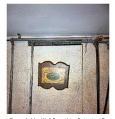
Figure 2-29. Wall Panel Has Detached From the Wall.
