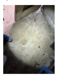
**Figure 4-36.** Drain Leads Directly Under the Foundation, Potentially Undermining the Foundation.
