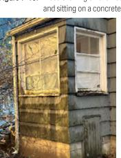
**Figure 7-21.** Moss on the Windowsills and Siding on Unit A's Back Entryway and Rot on the Windowsills.
