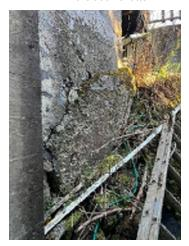
Figure 3-16. Cracked Concrete Wall/ Failed Foundation,
