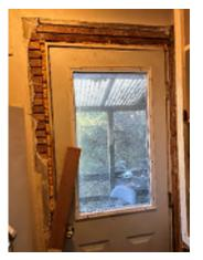
**Figure 3-26.** Damage to Plaster Around the Door because of Missing Trim.
