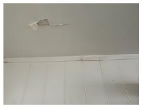
**Figure 4-19.** Peeled Paint With Signs of Water Damage on the Ceiling and Cracking in the Trim and Wallboards.
