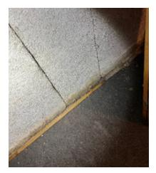
Figure 2-30. Bottom of the Wall Panel Has Water Damage.
