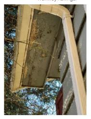
**Figure 7-24.** Deterioration to the Underside of the Eave.
