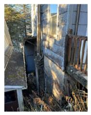
**Figure 3-13.** South Side of the Building and Rotten Deck.
