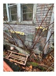
**Figure 4-4.** Siding Replaced With Roof Shingles and Spray Foam.
