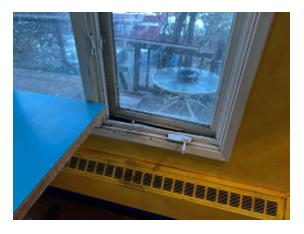
Figure 7-44. One Window No Longer Opens Properly.
