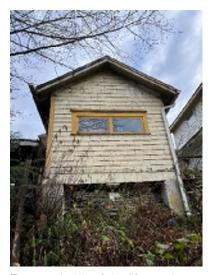
**Figure 5-16.** West Side of Garage. Paint on the siding has significantly deteriorated.
