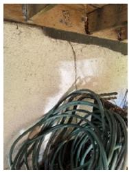
Figure 1-2. Large Concrete Crack on the South Wall.
