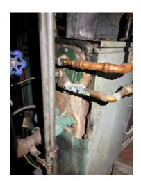
Figure 5-30. Significant Corrosion on the Boiler.
