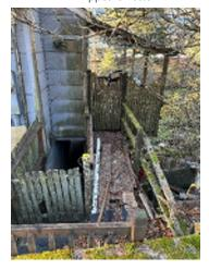
**Figure 3-4.** Rotten Gates, Railings, and Deck Framing Pose a Safety Hazard and Should Not Be Used.
