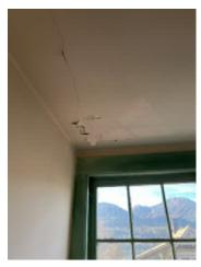
Figure 6-17. Cracking and Peeling Paint on the Ceiling.
