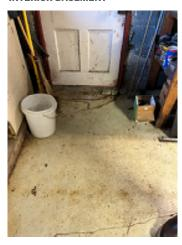
**Figure 6-22.** Cracked Slab-on-Grade at the North Basement Entrance.
