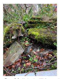
**Figure 5-8.** Undermined Walkway on the West Side of the Building.
