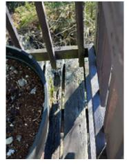
**Figure 7-40.** Rotten Boards on the corner of the Elevated Deck.
