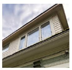
Figure 5-14. Moss on the Roof and Peeling Paint on the Eave.
