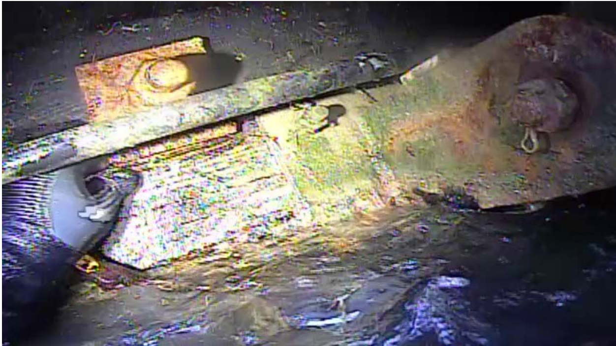
Image 2 – Inshore connection to bridge cracks located at diver's hand and below.
