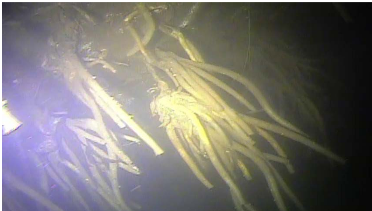
Image 2 – Light marine growth with tubeworms throughout the surface.
