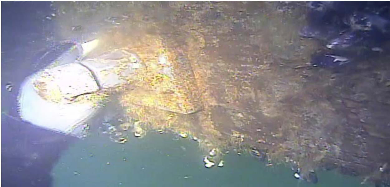
Figure 1 – Typical perimeter hardware, good condition and tight.
