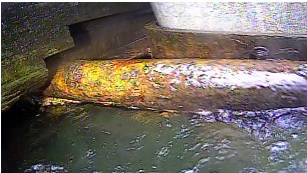
Image 3 – Standard piling hoop, corrosion and deflection noted
