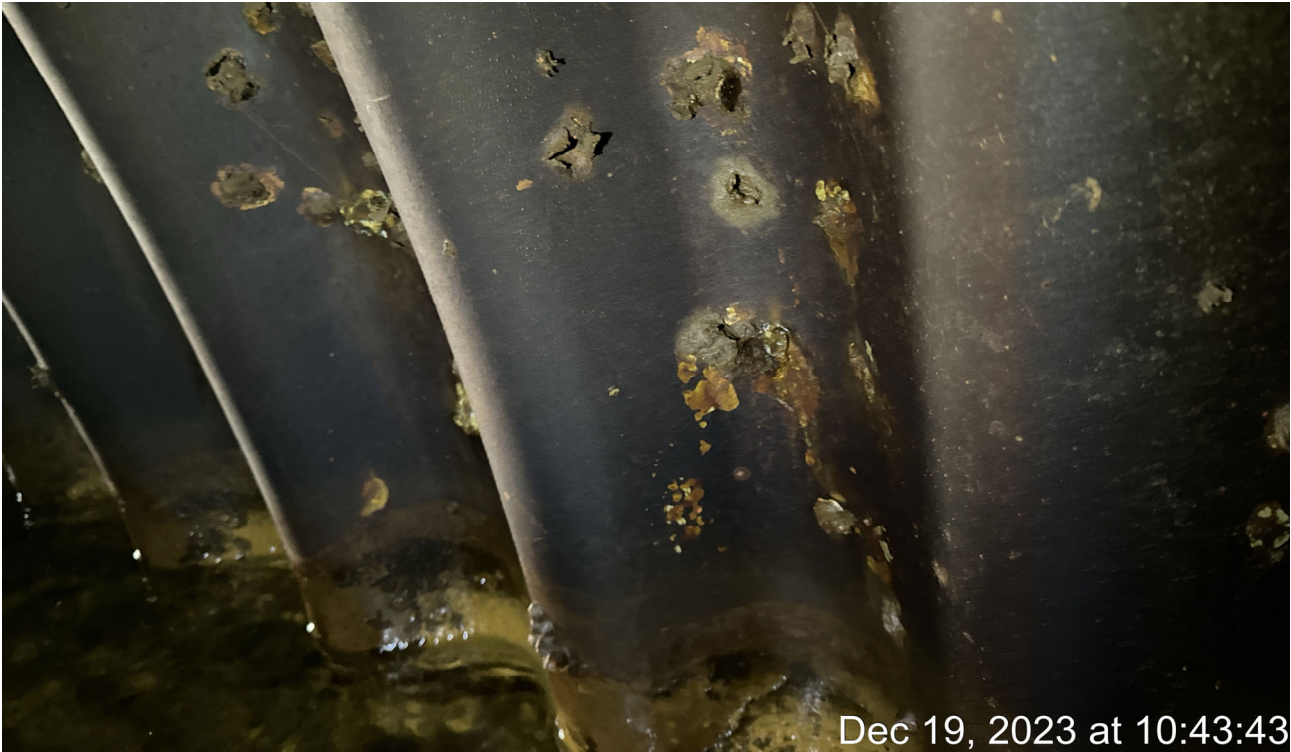
Photo 01: Heavy pitting and holes as observed on a portion of the half-arch culvert sidewalls.
