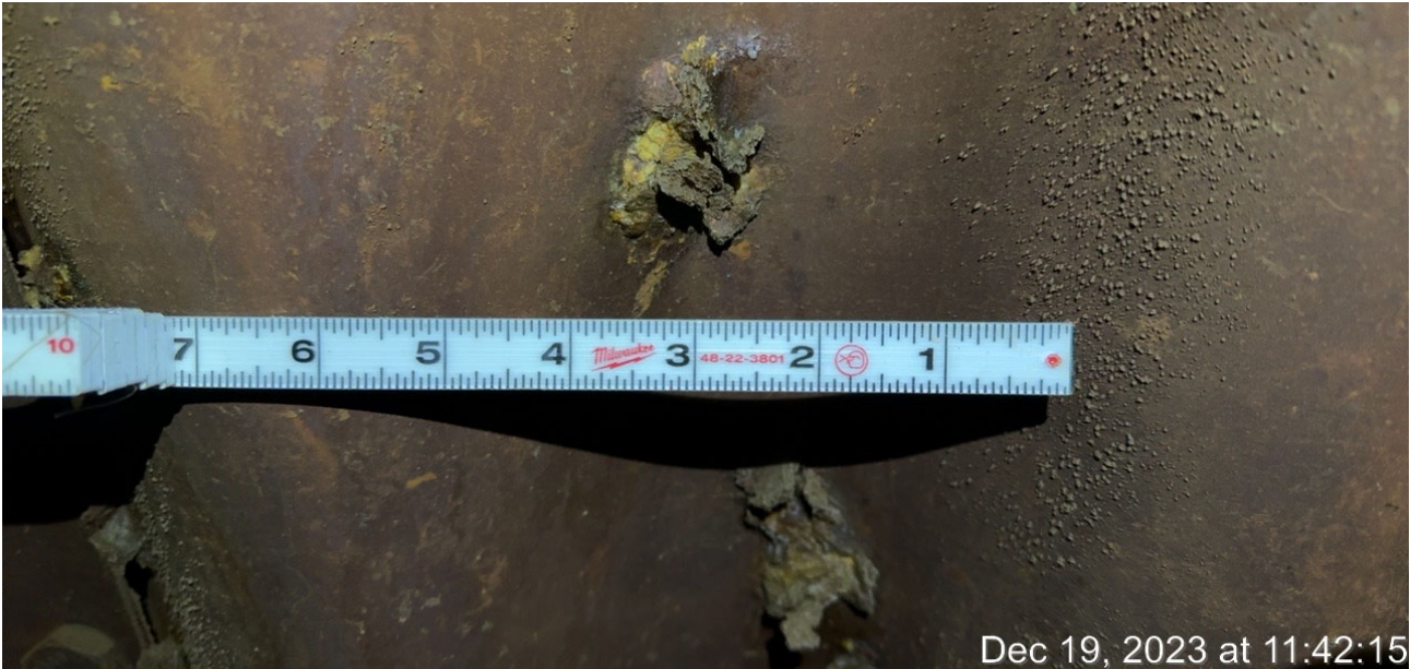
Photo 02: Holes in the culvert sidewall measure an inch in diameter or more.
