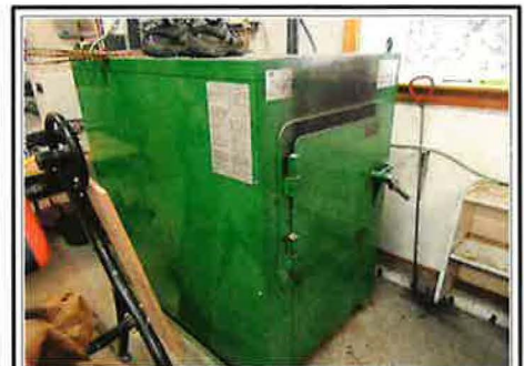
Wood and Oil Fired Boiler
