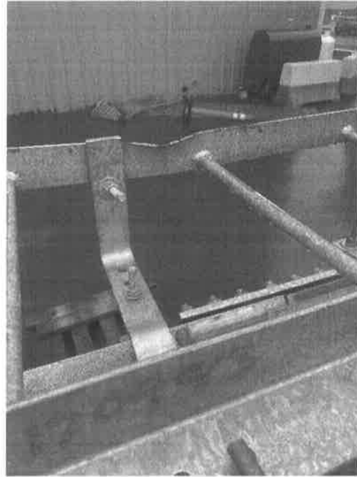
Photo 4 – (5/10/22) – Damage to one of the ladder sections.
