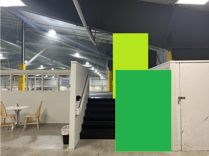
Proposed elevator stops on the mezzanine (green) and the track (lime green).
