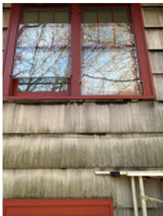
Figure 6-9. Deteriorating Window Sill.
