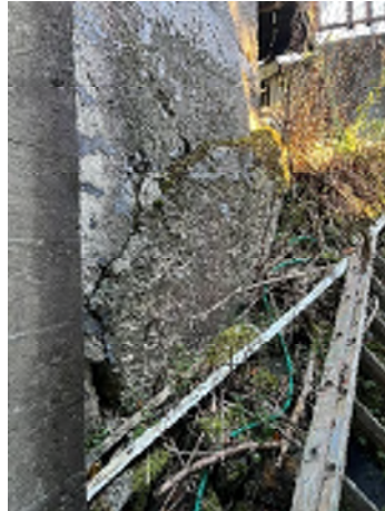
Figure 3-16. Cracked Concrete Wall/ Failed Foundation, Possibly From Flexure and Shifting. No reinforcement was observed. Collapse Hazard.
