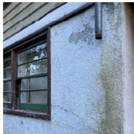
Figure 1-6. The Drainpipe Ends Abruptly in Mid-Air and Does Not Direct Water Away From the Foundation.
