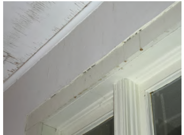
Figure 5-26. Indications of Water Damage on Windowsill.
