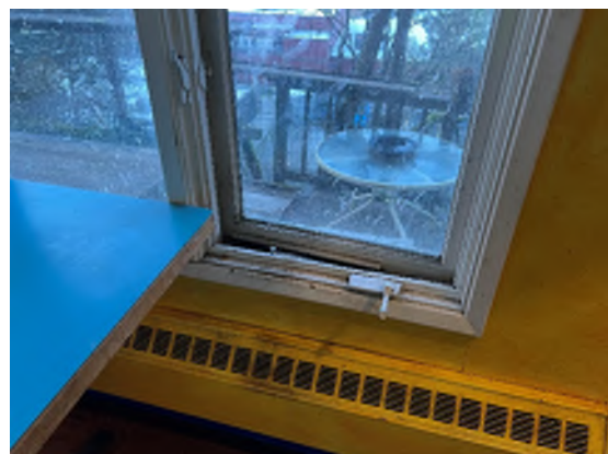
Figure 7-44. One Window No Longer Opens Properly.
