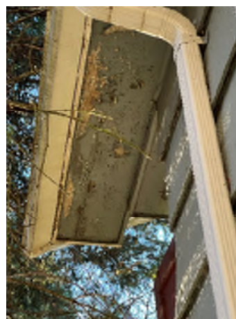
Figure 7-24. Deterioration to the Underside of the Eave.
