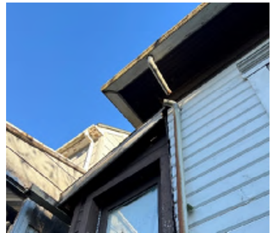
Figure 1-10. The Drainpipes Are Disconnected, and Water Is Not Directed Away From the Building.
