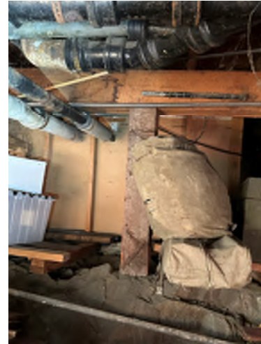
Figure 6-25. No Lateral Restraint/Connection From Beam to Column. The wood column is placed directly on top of the rock.
