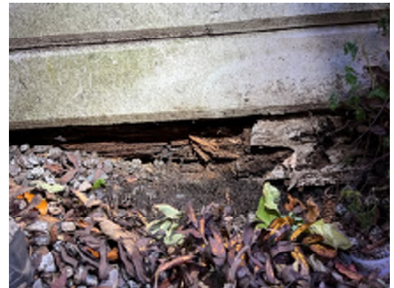
Figure 1-16. Exposed Wood Beneath the Siding Is Rotten.
