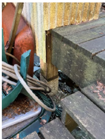
Figure 7-19. Moss Growing on the Deck. The column is shimmed and sitting on a concrete pile.
