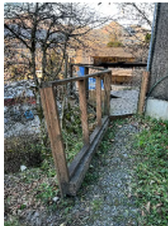
Figure 7-8. Leaning Handrails.
