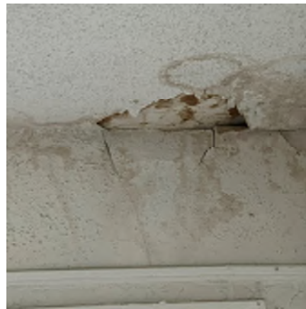
Figure 2-18. Ceiling Paint Is Cracked and Falling From the Wall Due to Water Infiltration. How extensive the water damage is or if there is mold is unknown without a destructive investigation.
