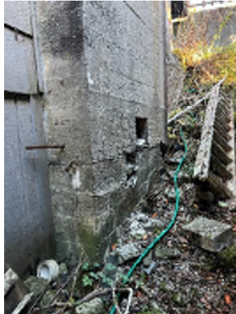
Figure 3-15. Failed Chimney Foundation Wall. Collapse Hazard.
