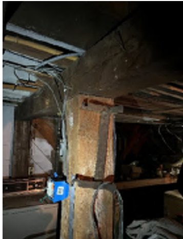
Figure 3-37. No Hardware Providing Connections from the Columns to Beam Above.
