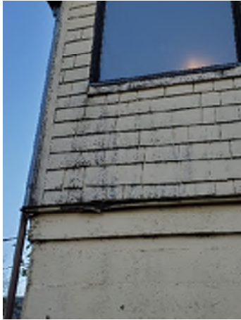
Figure 2-7. Black Mold on the Siding at the Southwest Corner.
