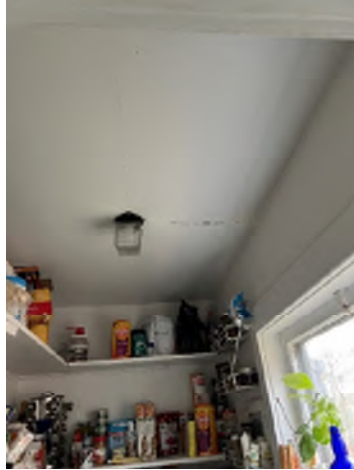
Figure 4-25. Sheetrock Cracks at Panel Edges.
