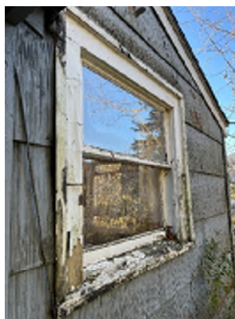
Figure 3-10. Rotten Windowsill and Siding in Poor Condition.
