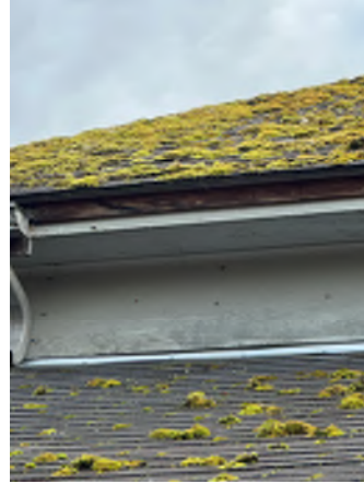
Figure 4-2. Exposed, Rotting Wood on the Eave.
