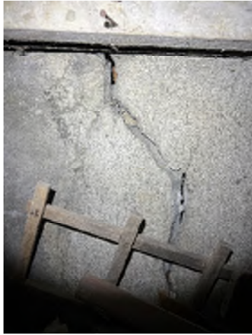
Figure 1-13. Visible Wood Framing in the Deep Crack Where Water Infiltrates the Basement.
