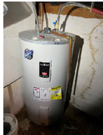
Figure 2-36. No Seismic Strapping Around the Water Heater.
