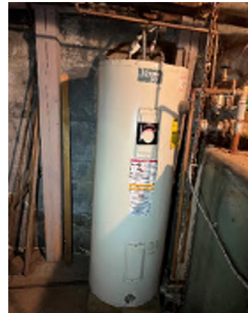
Figure 3-40. No Seismic Strapping Around the Water Heater.
