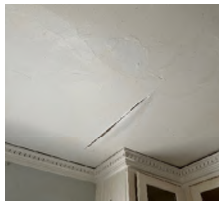
Figure 3-24. Sheetrock Cracks and Water Damage on the Ceiling.
