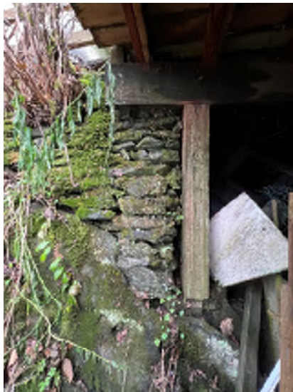
Figure 5-11. Column is Sitting on a Rock.
