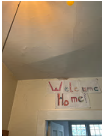
Figure 6-20. Cracked Drywall and Drooping Ceiling.
