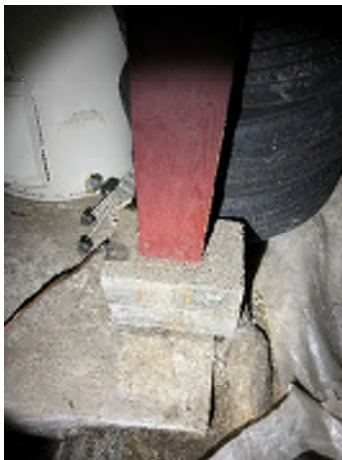
Figure 7-50. The Column Is on a Concrete Block That Is Not Sitting Fully on the Concrete Below.
