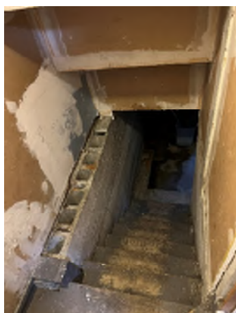
Figure 7-45. No Grout Columns Were Observed in the Visible Portion of the Masonry Wall. This wall is likely unreinforced.
