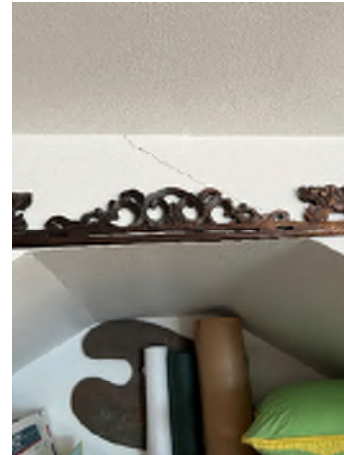
Figure 7-36. Sheetrock Cracks Through the Unit.
