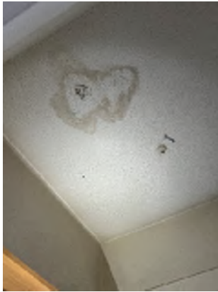
Figure 2-23. Water Damage, Cracks, and Exposed Wiring in the Closet on the Northeast Side of the Building.
