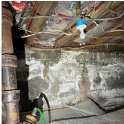
Figure 1-27. Many Signs of Water Infiltration Exist on this Concrete Wall From the Discoloration. The sill plate is rotten from the outside.
