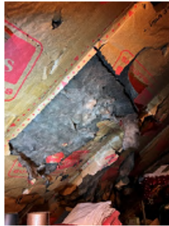
Figure 7-38. Paper Came off the Insulation, and the Insulation Corners Are Falling in the Attic Space.
