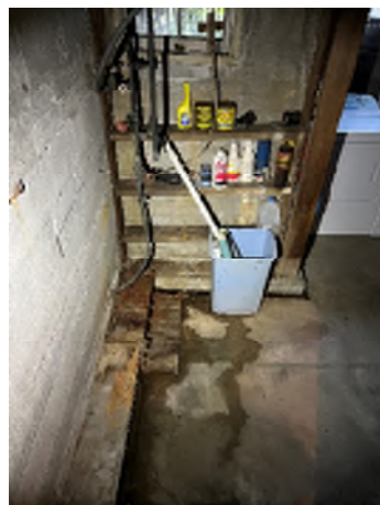
Figure 7-47. Multiple Signs of Water on the Basement Floor. There is a small trench for water around the perimeter.
