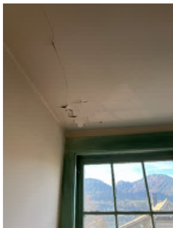
Figure 6-17. Cracking and Peeling Paint on the Ceiling.
