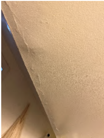
Figure 7-37. Paint Is Chipped, and the Sheetrock Fasteners Are Visible in Some Places.
