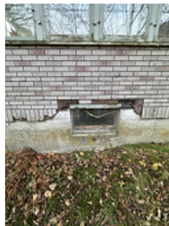
Figure 4-6. Deteriorated Siding and Windowsills.
