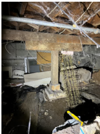
Figure 4-35. Column Sitting Directly on the Foundation With No Positive Connection to the Concrete or to the Beam.
