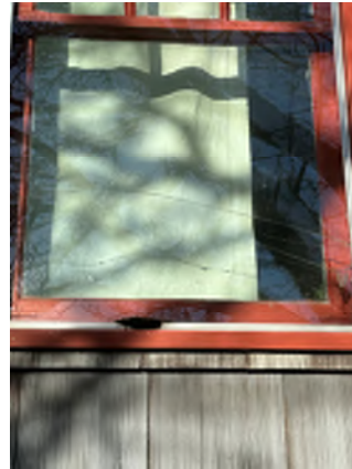
Figure 6-14. Crack in the Storm Window.
