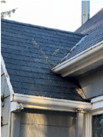
Figure 3-3. Plant Growth Indicates Build-up in Gutter.
