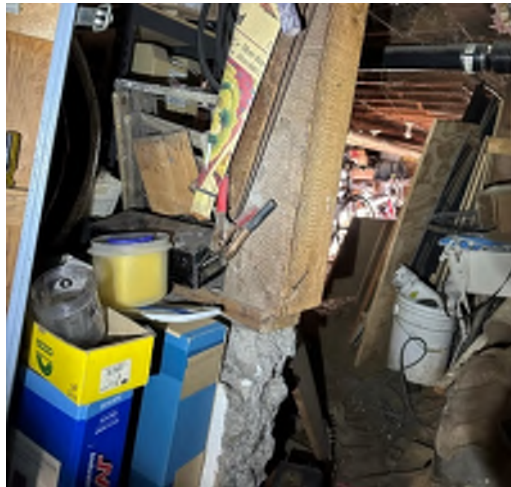
Figure 6-24. Wood Post Supported Eccentrically by Stem Wall With a Chunk of Concrete Missing Directly Below the Post.
