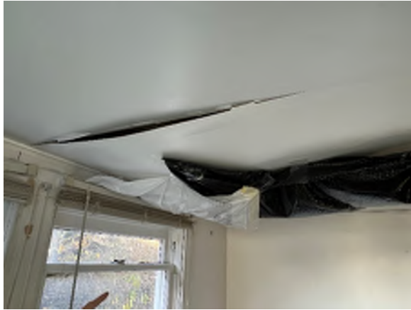
Figure 3-31. Ceiling Damage From a Roof Leak.
