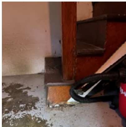
Figure 1-27. Many Signs of Water Infiltration Exist on this Concrete Wall From the Discoloration. The sill plate is rotten from the outside.
