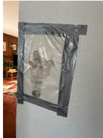
Figure 7-34. Mold Is Growing Under the Vapor Barrier. The Extent of Damage in the Wall Cavity Is Unknown.
