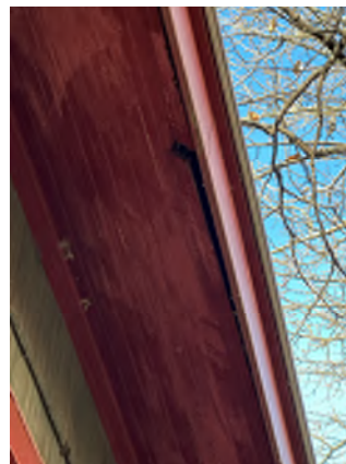
Figure 6-10. Damaged Eave.
