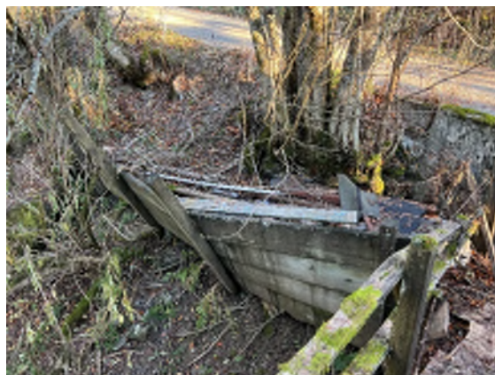
Figure 3-8. Failed Wooden Retaining Wall.
