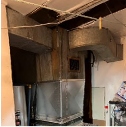
Figure 1-25. Staining on the Ducting Indicating Past Leaks.
