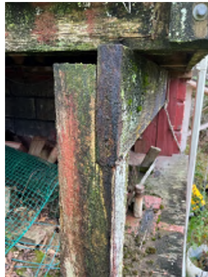
Figure 5-12. Rotten Beam Support and Deck.
