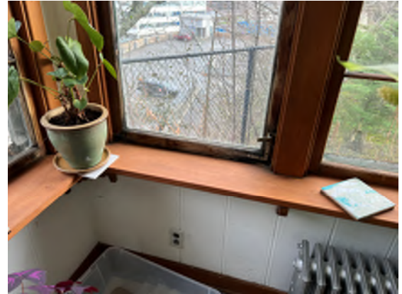
Figure 4-20. Rotting Window Frame.
