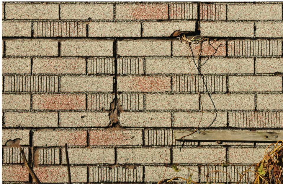
Asphalt-shingle siding covers the original clapboard siding. Therefore the residence does not retain the key exterior materials dating from the period of its historic significance. Edward Webster House, 2023
