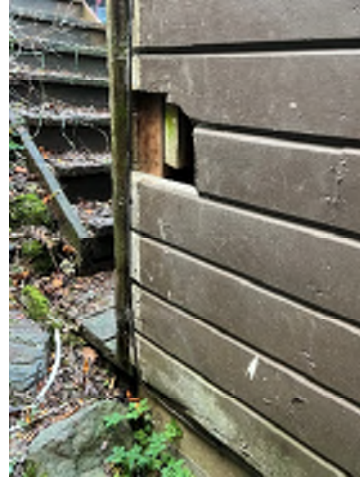
Figure 1-14. A Hole in the Siding That Can Allow Water or Animals in the Wall Cavity.
