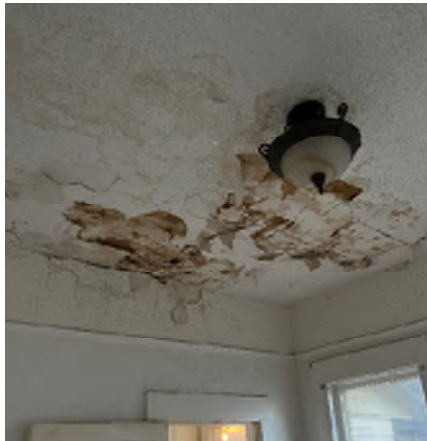
Figure 2-17. Significant Water Damage to the Ceiling Below the Roof Leak. The light fixture was not tested because of signs of water infiltration.
