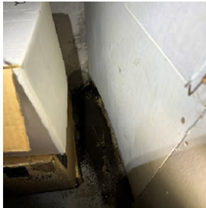
Figure 1-30. Channel Under the Stairs Where Water Frequently Flows In. This is the location of the large concrete crack on the north side wall.
