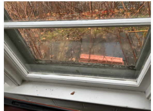
Figure 4-22. Rotting Storm Window and Window Frame.
