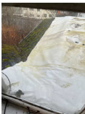
Figure 4-11. Tarp Covering the East Roof. There are known leak issues at the interface of the lower roof and wall.
