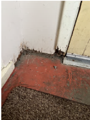
Figure 5-25. Rotting Wood Next to the Entryway Door.
