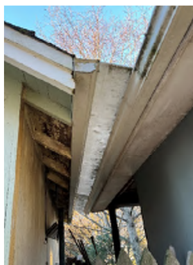
Figure 5-18. Deterioration Under the Eave.
