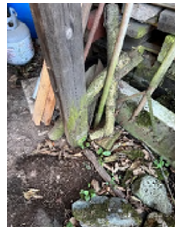
Figure 7-28. Moss Growing on Main Column Supports That Are not Pressure Treated. These columns can rot quicker untreated.
