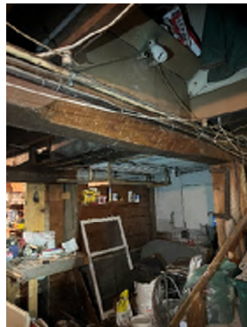
Figure 3-42. Notched Large Beam at the Bottom of the Stairs to prevent head injury.
