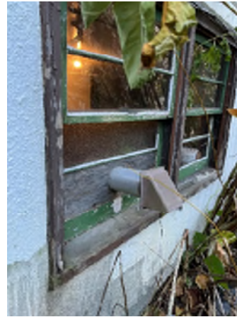
Figure 1-8. Rotten Window Sill.
