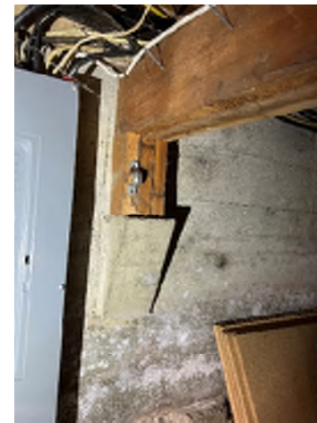
Figure 4-34. Nonstandard Beam Support.
