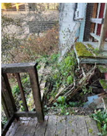
Figure 7-11. Moss on the Stair Landing and a Pile of Wood on the Ground.
