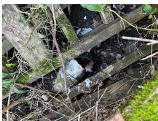
Figure 7-12. A Broken Pipe Below the Pile of Wood That May Be a Sewer Pipe.
