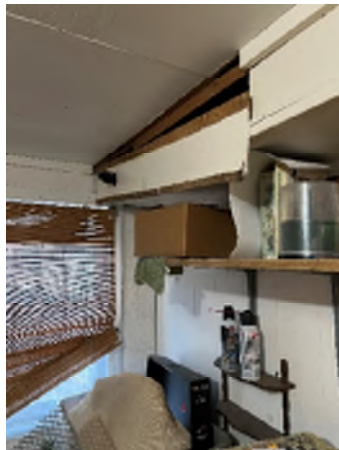
Figure 2-27. Wall Finishes Have Detached.
