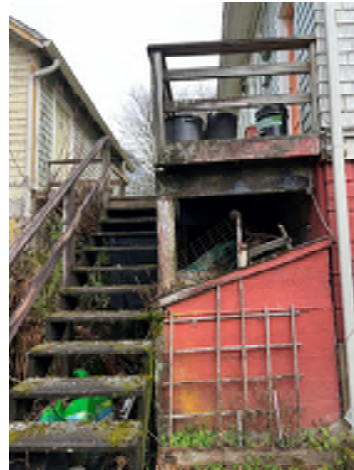
Figure 5-10. Rotted Deck and Stairs. Deck posts are not anchored and have no positive connection to joists.
