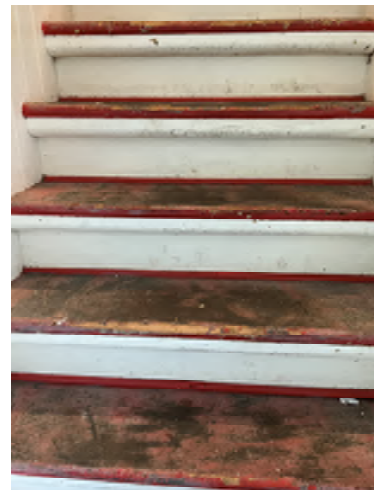
Figure 4-18. Steps Leading to the Second Floor Are in Poor Shape.
