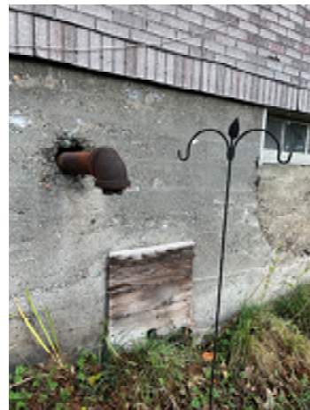
Figure 4-10. Large Hole Where Pipe Exits the Basement and Cracking Between the Different Concrete Pours Under Window.
