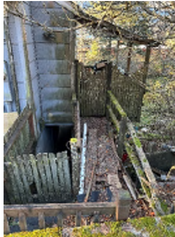
Figure 3-4. Rotten Gates, Railings, and Deck Framing Pose a Safety Hazard and Should Not Be Used.
