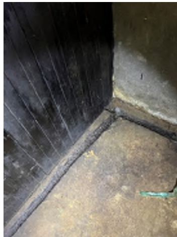
Figure 4-33. Trench Around the Perimeter for Water Flow.
