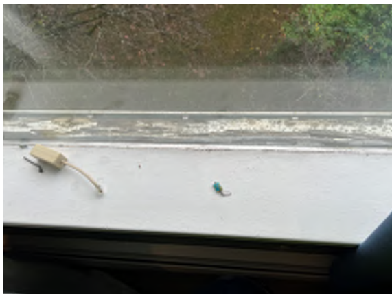
Figure 5-23. Deteriorating Windowsill.
