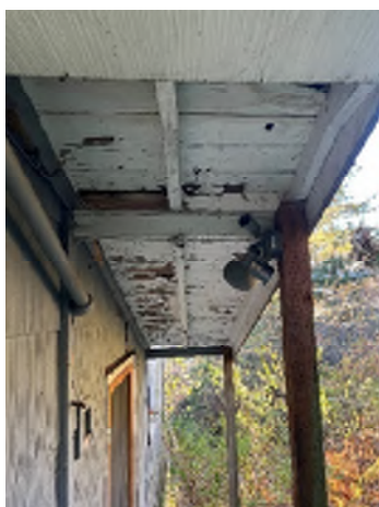
Figure 3-9. Peeling Paint and Fixtures Missing Bulbs; Open Fixtures or Exposed Wiring Can Be Hazardous.
