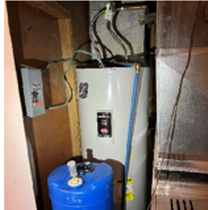
Figure 1-26. Water Heater Without Seismic Strapping.
