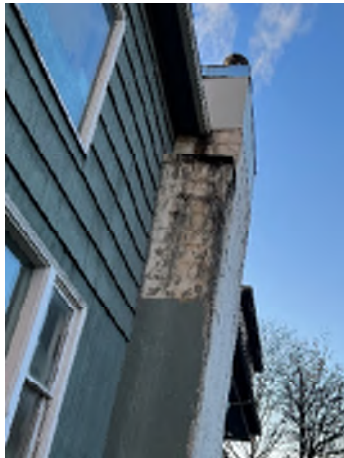
Figure 7-15. Water-Stained Chimney With Visible Cracks.
