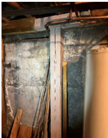
Figure 3-39. Significant Checking in this Column.
