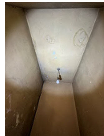
Figure 4-30. Cracking on the Ceilings and Walls and Signs of Water Damage.
