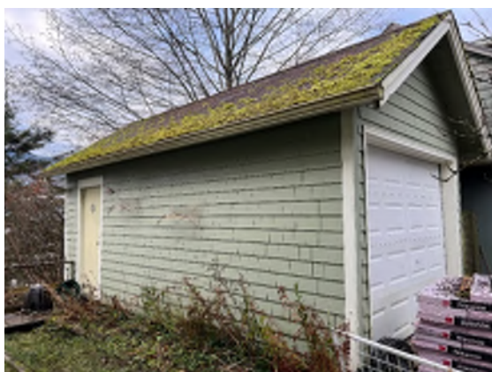
Figure 5-13. North Side of the Building. No Shear Wall / Lateral System on Front on Garage.
