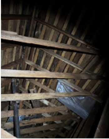
Figure 2-13. Attic Trusses and Most of the Wood Appears Dry. The roof rafters and site built trusses are under sized for current snow loads.
