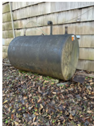
Figure 6-8. Fuel Tank Is Not Seismically Anchored.
