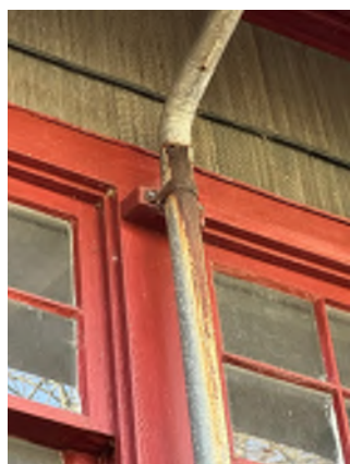
Figure 6-11. Drainpipe Is Rusted.
