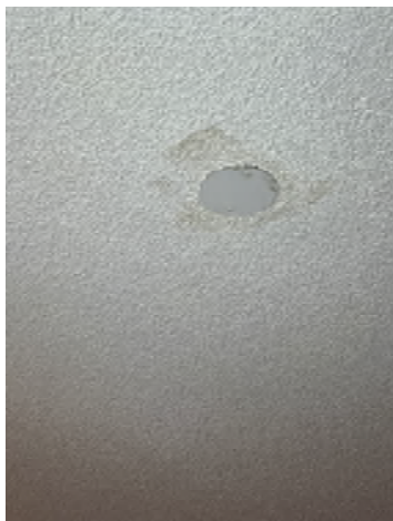
Figure 5-27. Water Damage Around Light Wiring Cover.
