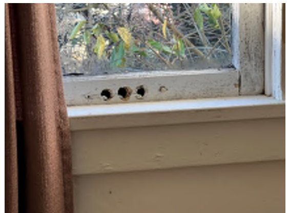
Figure 3-34. Mold and Holes in the Windowsill. The holes can lead to water infiltration.
