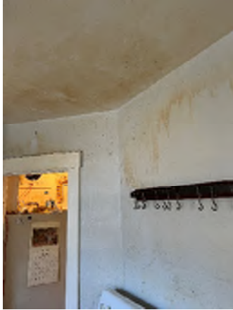
Figure 3-25. A Significant Amount of Discoloration on the Sheetrock Above the Stove in the Kitchen, Water Damage.
