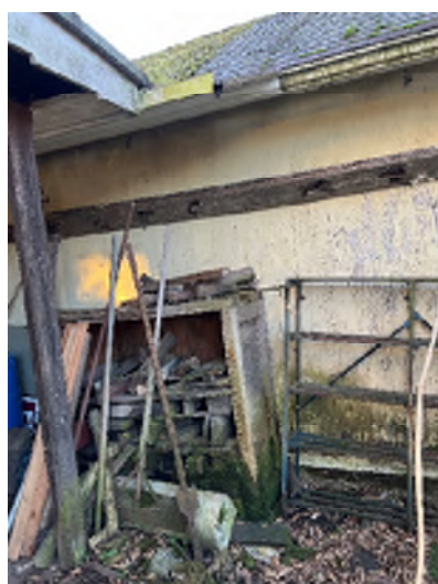
Figure 5-17. Gutter Drainage Splashed on the Garage and Caused Significant Moss to Grow and the Plywood to Rot.
