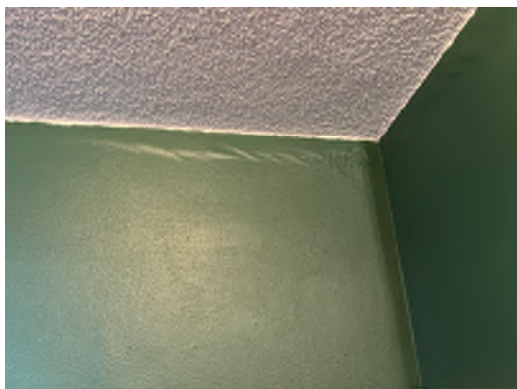
Figure 5-21. Bubbled Paint.
