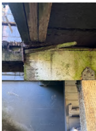
Figure 3-6. The Beam Supporting the Deck Is Shimmed Likely Due to Rot. No connection exists between the beam to deck framing.
