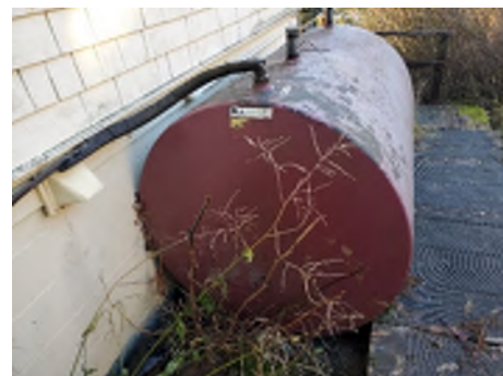
Figure 2-12. Tank Is Not Seismically Anchored.
