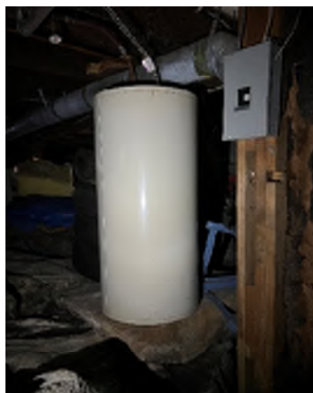
Figure 7-52. The Tank Is Not Seismically Secured.
