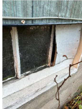
Figure 7-16. A Basement Broken Window, Which Is Not Adequately Sealed, That Can Allow Water or Animals Inside.
