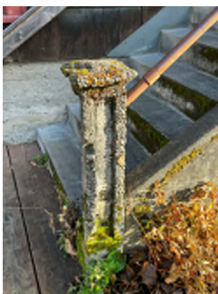
Figure 6-3. Damaged Concrete Post.
