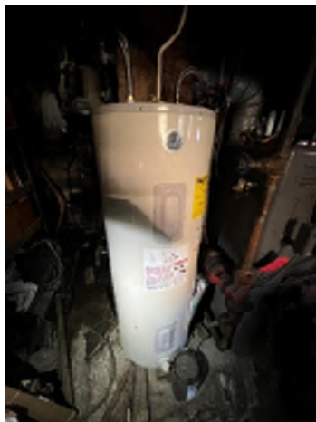
Figure 6-26. No Seismic Strapping on the Water Heater.
