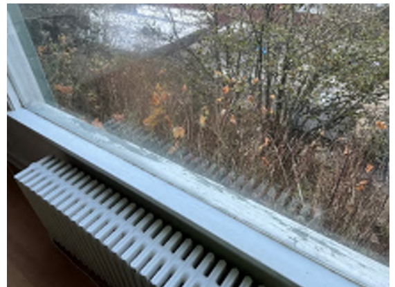
Figure 7-42. The Window Frame Has Some Deterioration.
