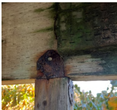
Figure 1-3. Rusty Hardware Connections on the Deck Framing.
