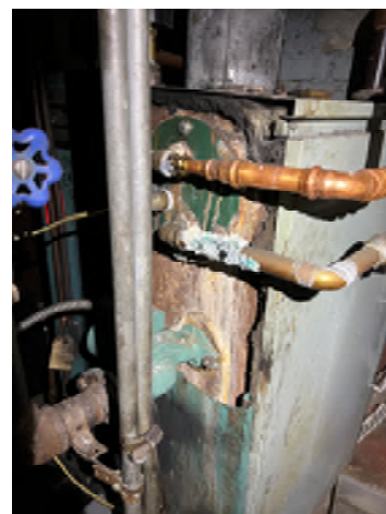
Figure 5-30. Significant Corrosion on the Boiler.
