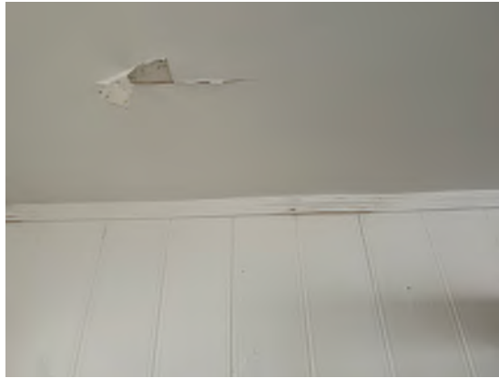
Figure 4-19. Peeled Paint With Signs of Water Damage on the Ceiling and Cracking in the Trim and Wallboards.
