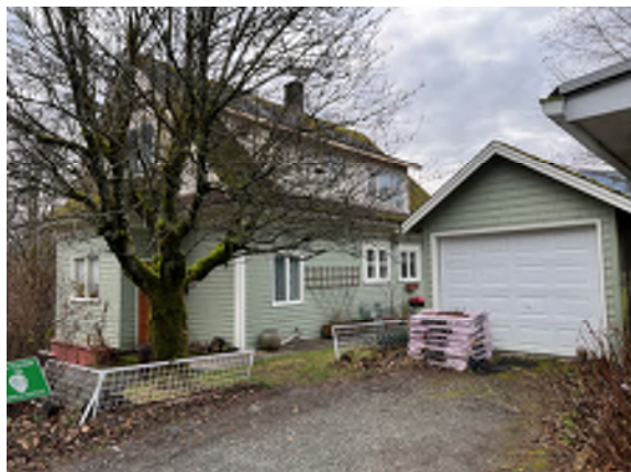
Figure 5-13. North Side of the Building. No Shear Wall / Lateral System on Front on Garage.
