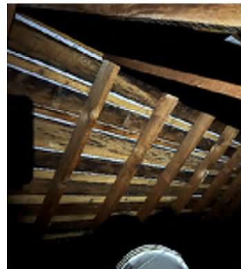
Figure 2-16. Indications of Previous Leak Repairs. Water infiltration can cause the structural members to rot. The roof rafters and site built trusses are under sized for current snow loads.
