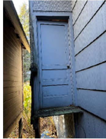
Figure 3-14. A Door Without Stairs Approximately 6 Feet Above the Ground. Some of the framing around the door is rotten.
