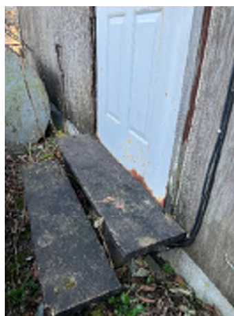
Figure 7-6. Unprotected Plywood Sheathing by the Siding and Rust Around the Man Door.
