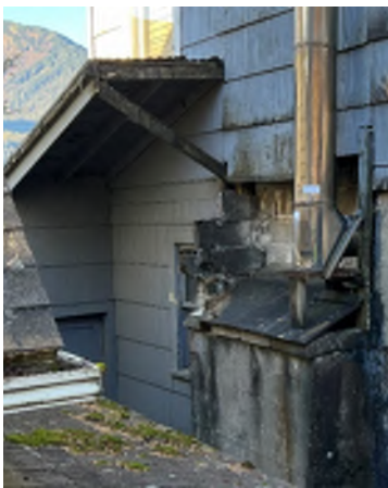
Figure 3-18. Concrete Blocks Not Adequately Secured. The new stack is partially supported on a rotten piece of plywood.
