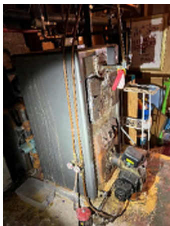
Figure 2-33. Signs of Leaks Exist With the Staining on the Side of the Unit.
