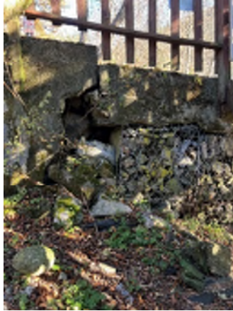
Figure 1-19. Undermining of the Road at the Interface Between the Two Retaining Wall Systems.
