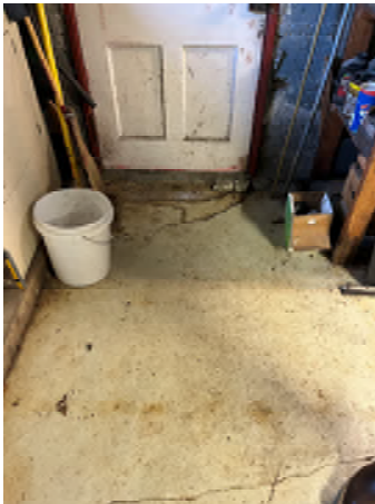
Figure 6-22. Cracked Slab-on-Grade at the North Basement Entrance.
