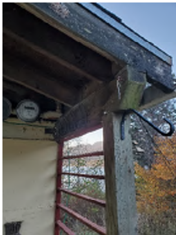
Figure 2-3. Roof Members on the Canopy Appear Rotten. No uplift connection exists between the post and beam.
