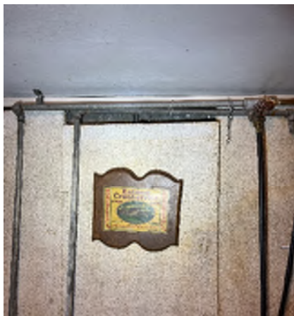
Figure 2-29. Wall Panel Has Detached From the Wall.
