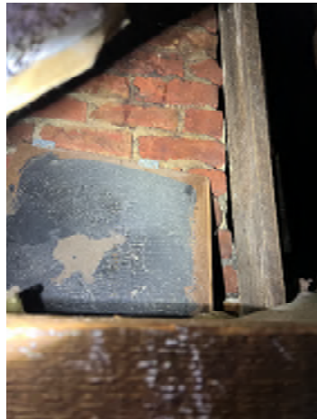
Figure 5-20. Deteriorating Chimney.
