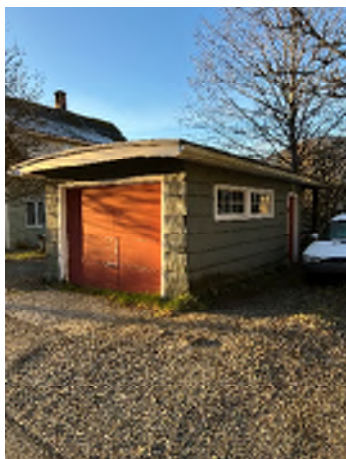
Figure 7-25. Garage/Shed on the South Side of the Building. No Lateral System on Front.
