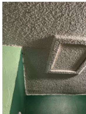
Figure 5-22. Cracked Ceiling Drywall.
