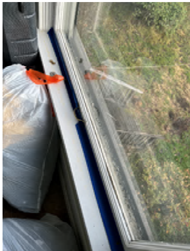
Figure 4-17. Deteriorating Windowsill.
