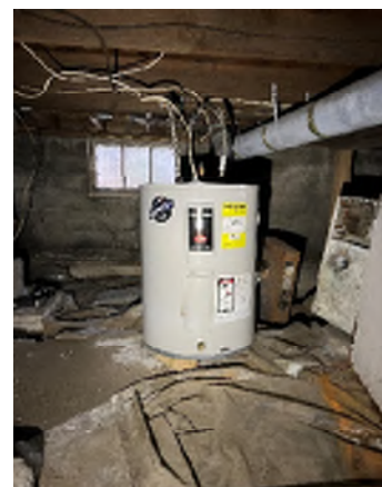
Figure 7-53. The Tank Is Not Seismically Secured.
