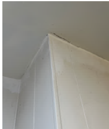
Figure 5-24. Continuous Ceiling Crack Around a Corner.
