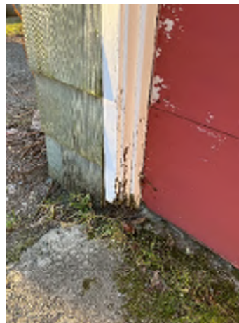
Figure 7-26. Rot Near the Ground.
