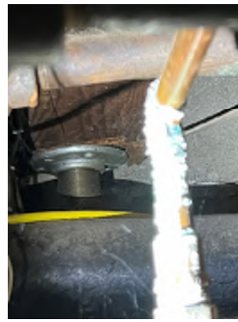
Figure 2-38. A Pipe Supporting a Beam With No Positive Connections at the Top or Base.
