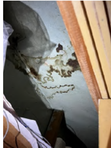
Figure 4-26. Staining on Ceiling.
