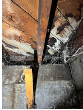
Figure 4-32. Rotting Floorboards.
