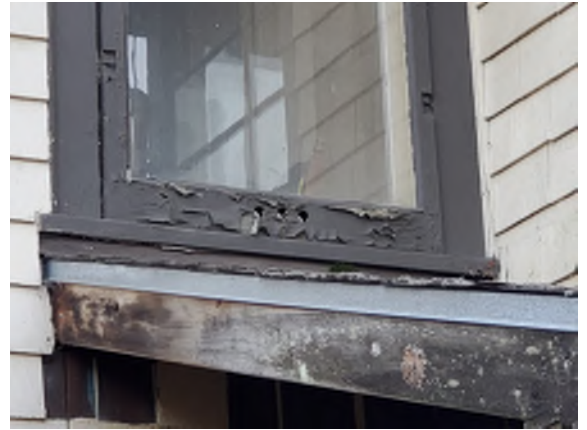
Figure 2-2. Three Holes in the Window That Could Allow Water to Enter the Building.
