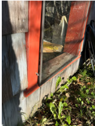
Figure 6-13. Gap in the Storm Window.
