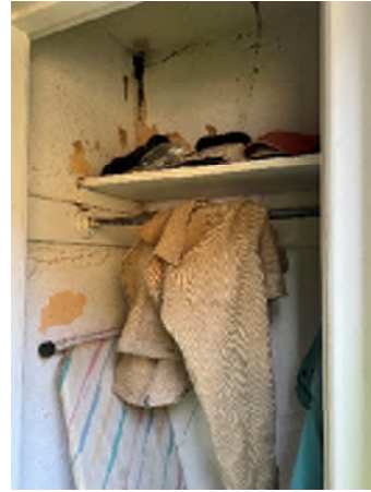
Figure 3-20. Significant Sheetrock Damage in the Closet.
