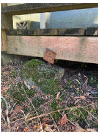
Figure 7-23. A Rotated Walkway Support Connector.
