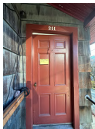
Figure 6-4. Large Gap Between the Door and Doorframe.
