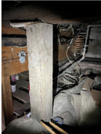
Figure 7-48. One Column Is Sitting on the Bedrock With No Connections. There are shims at the top of the column.
