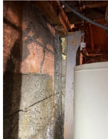
Figure 3-38. No Positive Connection From this Column to the Beam Above and the Column Has Shifted.
