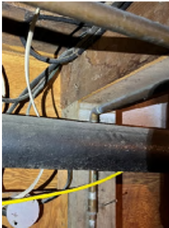
Figure 2-37. Columns Are Toe-Nailed at the Top to the Beam. No positive connection at the base of the column to the concrete exists.
