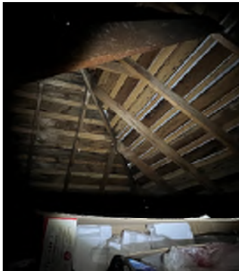
Figure 2-15. Daylight Is Visible Through Holes in the Northwest Corner of the Roof, Which Allows Water to Penetrate the Roof. This is the cause of the water damage seen on the ceiling of the second level. A roof replacement is in progress.
