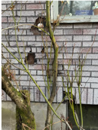
Figure 4-3. Holes in the Siding.
