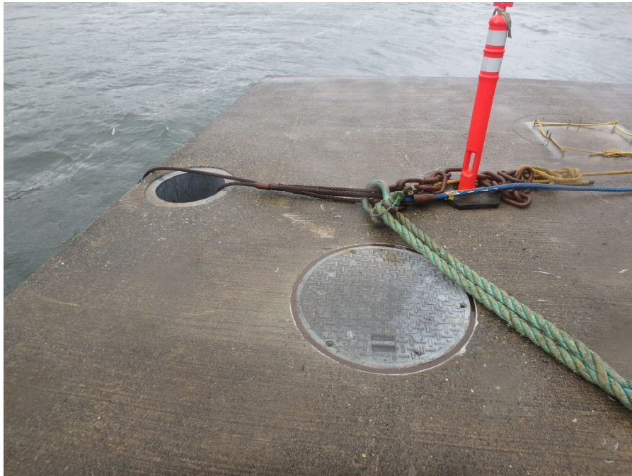
Photo 7. Hawse pipe and water tight manhole cover
