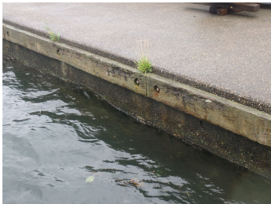
Photo 10. Worn timber rubboards with vegetation.
