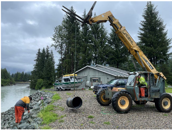
Figure 2 Image of installation of check valve at Rivercourt Way.
