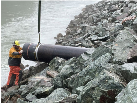
Figure 3 Image of installation of check valve at Rivercourt Way.
