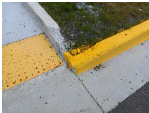
PHOTO 06: Damage at one of the accessible ramps.
