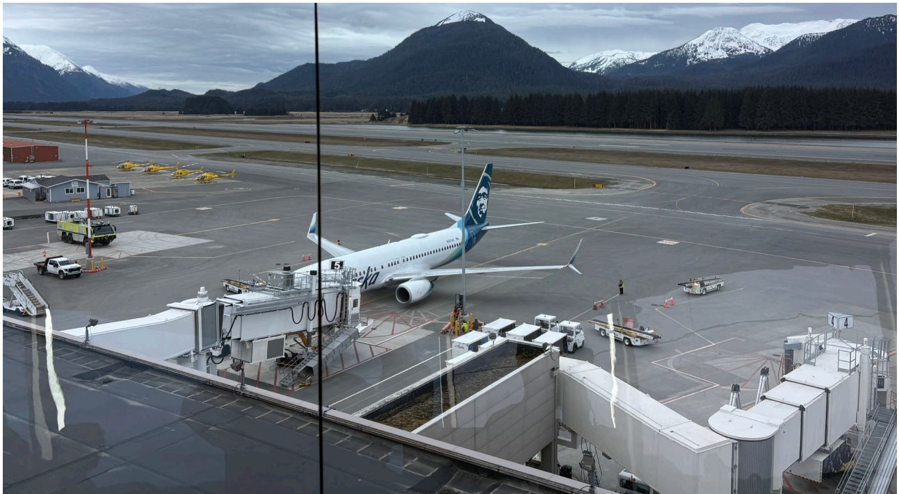
Light Pole LP-4 (on the right) and LP-5 (on the left). LP-4 is approximately 204 feet from the cab. LP-5 (striped) is approximately 320 feet from the cab. Both assemblies are 57.5 feet tall.
