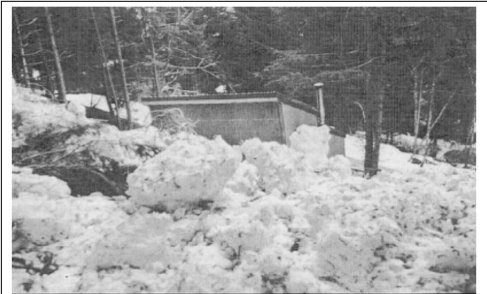
White Subdivision residence after avalanche of February 20, 1985. Only the second story is visible above the avalanche debris. Photo by Doug Fesler.
