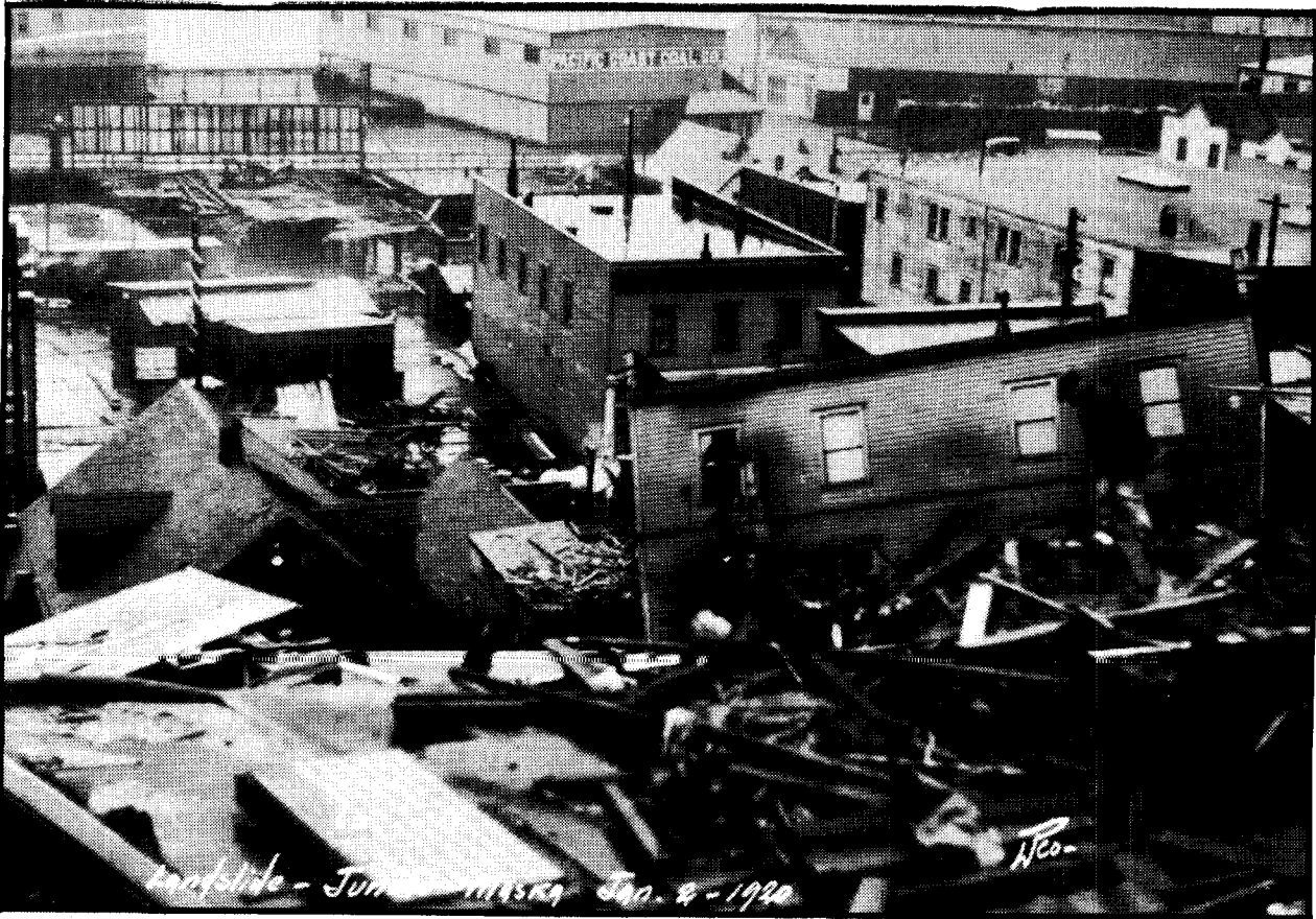
Figure 3. This view of the area between Gastineau Ave. and S. Franklin St. (Jan. 2, 1920) illustrates how buildings were destroyed by a debris avalanches through the processes of impact and relocation. Source: Alaska Historical Library, Early Prints of Alaska Collection.
