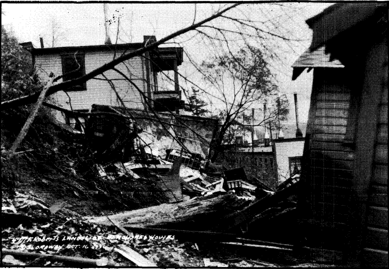
Figure 4. This debris avalanche on Oct. 16, 1936 destroyed buildings between Gastineau Ave. and S. Franklin St. by crushing and relocation. Source: Alaska Historical Library, Early Prints of Alaska Collection.
