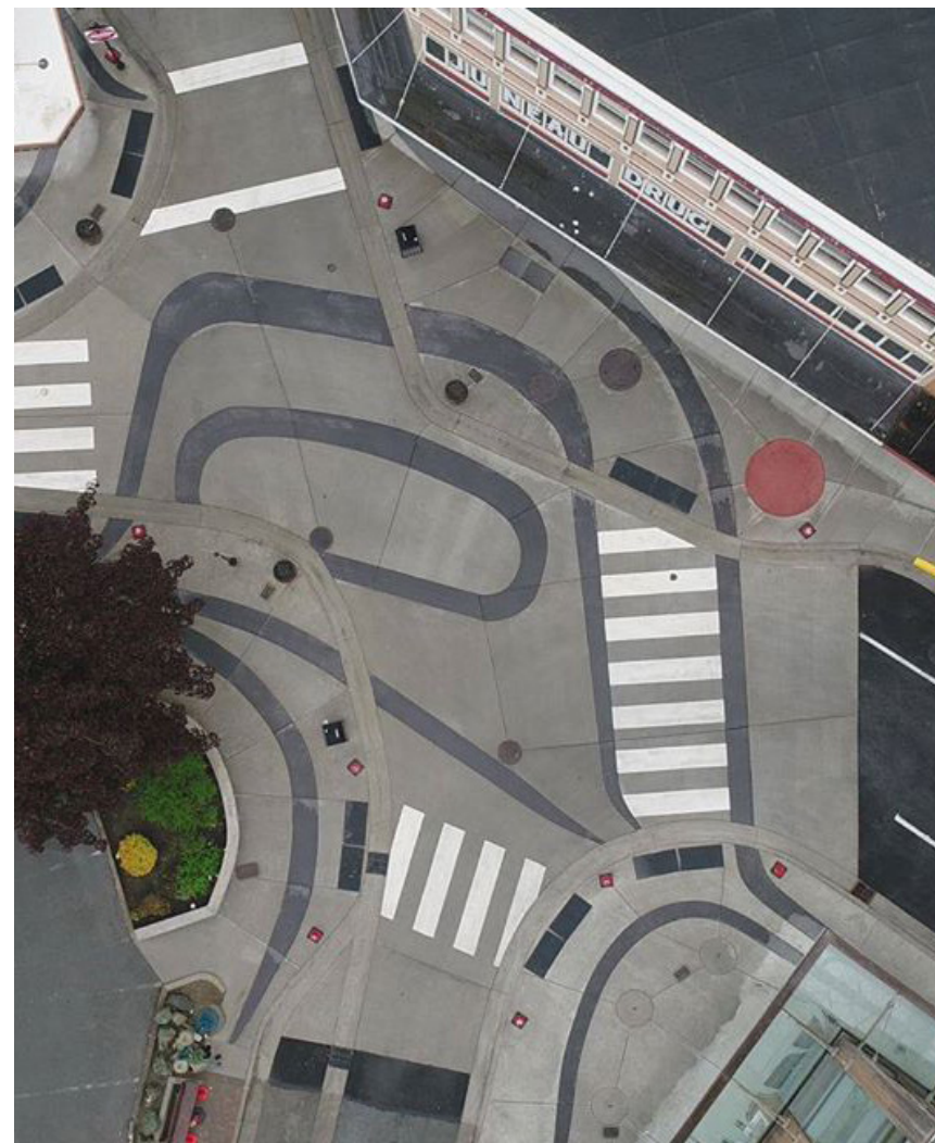
Photo Credit: CBJ General Engineering
