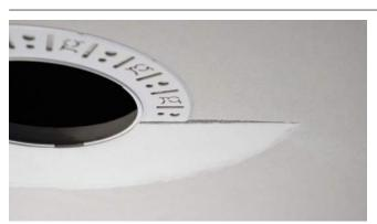
Partially finished mud ring, showing cross-section detail.
