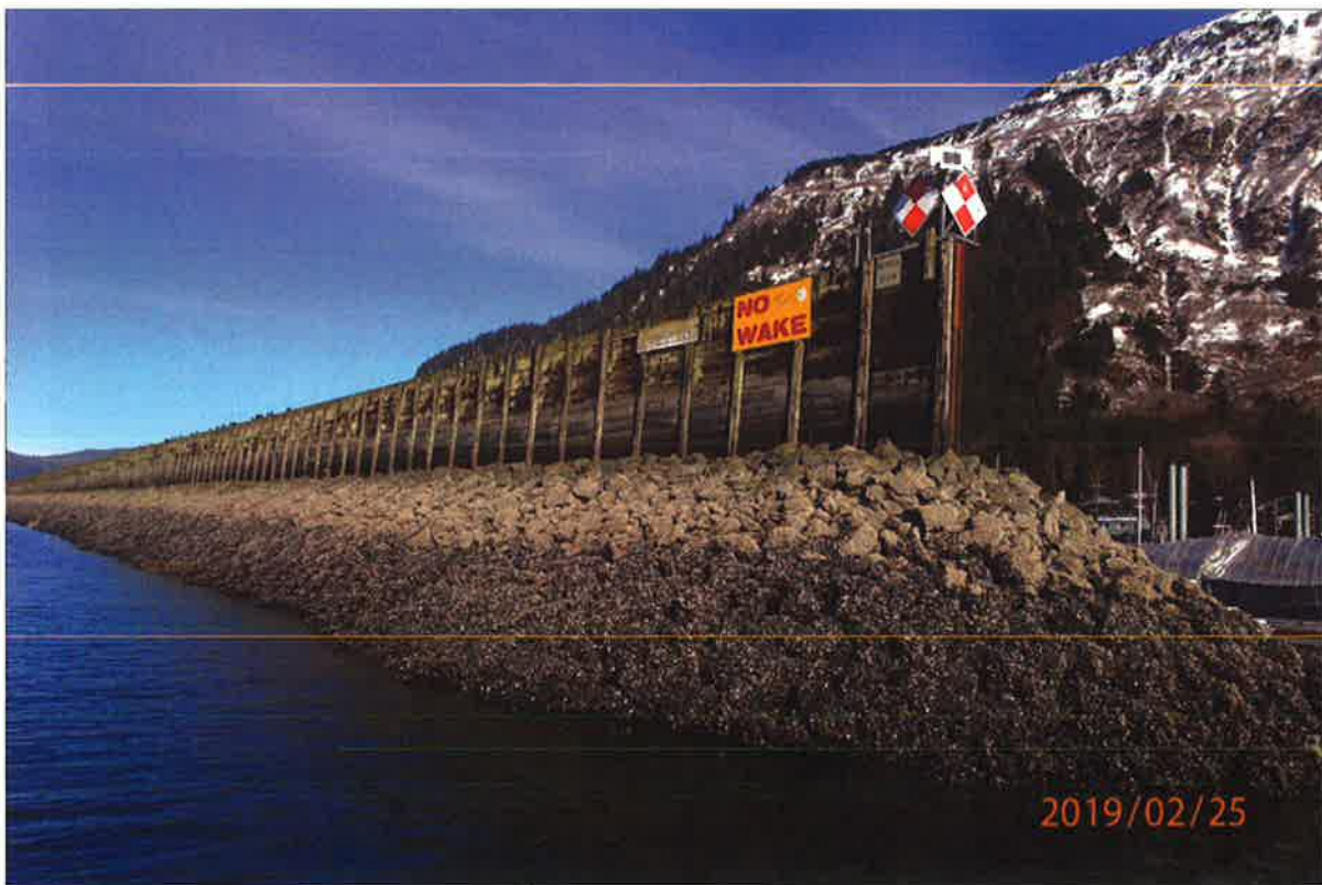
Figure 11. Composite wave barrier at Aurora Harbor, Juneau (USACE 2019).
