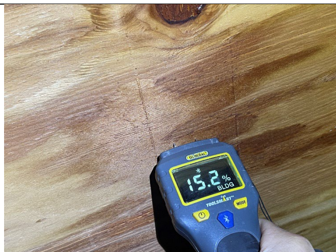
Aurora Harbor Office: Many areas of underside of roof deck have active water intrusion and high moisture levels.
