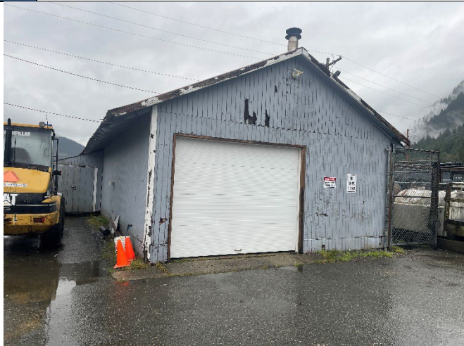
Aurora Harbor Outbuilding/Garage: General view of West side of building. In general the building has outlived its useful life and is heavily water damaged. The exterior envelope has many signs of water damage and wood decay. The structure does not meet accessibility requirements.
