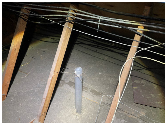
Aurora Harbor Office: View of unconnected exhaust fan from main entry office into attic space.
