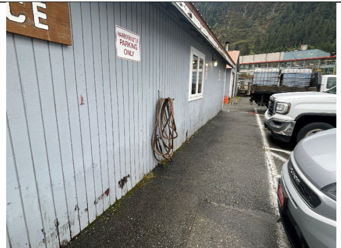
Aurora Harbor Office: Wood decay along base of siding. Appurtenances along face of structure sticking out into accessible aisle.
