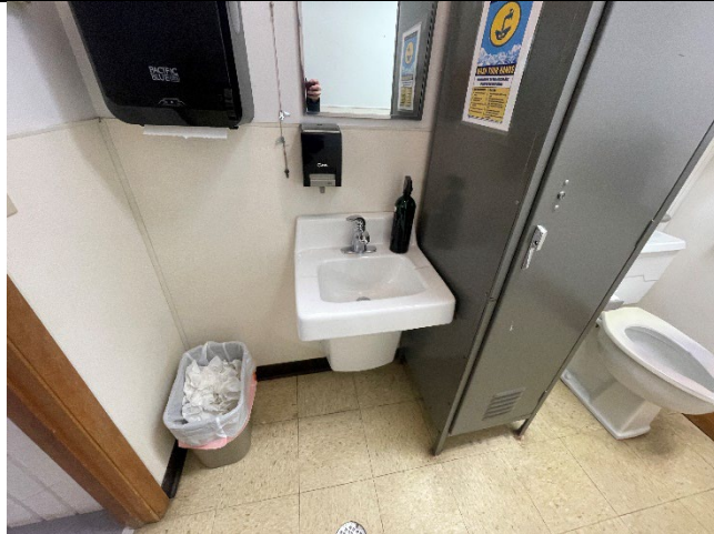
Aurora Harbor Office: South bathrooms off of the front main office does not meet accessibility requirements at toilet and lav.
