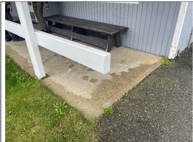
Aurora Harbor Office: Asphalt paving and concrete sidewalk not aligned and is a tripping and accessibility hazard.
