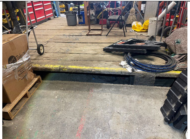
Aurora Harbor Outbuilding/Garage: General view of interior floor transitions at Outbuilding interior. Area does not meet accessibility requirements.
