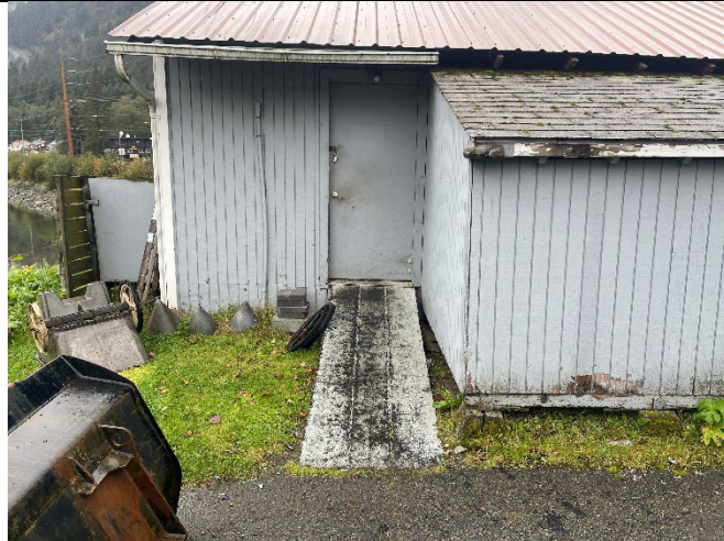
Aurora Harbor Outbuilding/Garage: General view of Southwest door. Access does not meet accessibility requirements.
