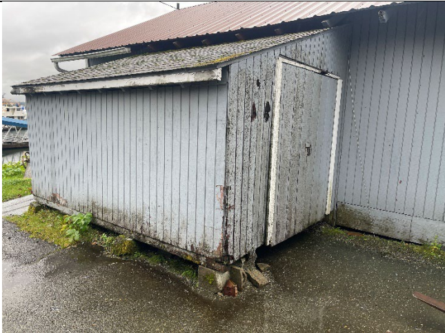
Aurora Harbor Outbuilding/Garage: General view of water damaged and decay.
