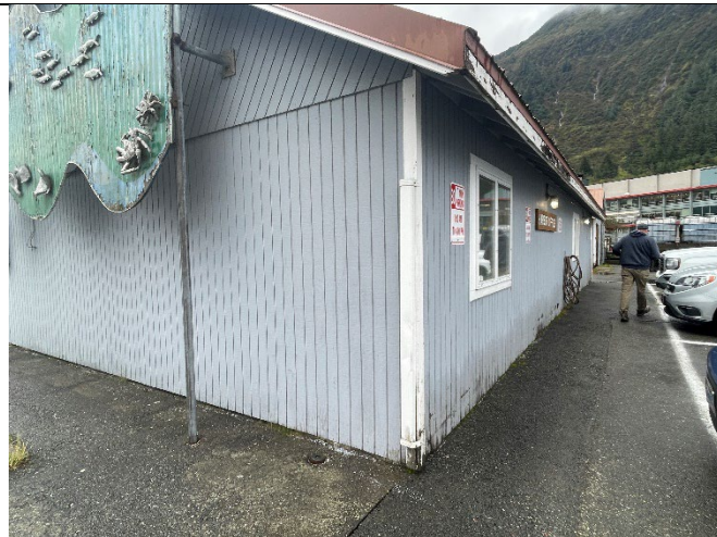
Aurora Harbor Office: Missing gutters has contributed to trim and siding water damage and wood decay.
