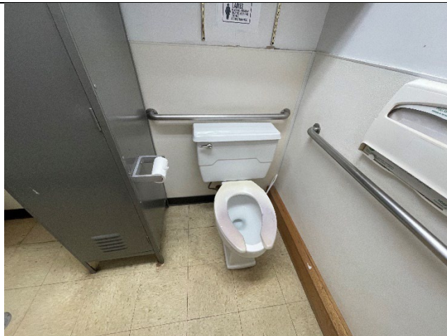
Aurora Harbor Office: South bathroom water damage at wall from broken vent pipe through the roof. Enlarged view of South bathrooms not meeting accessibility requirements at toilet.
