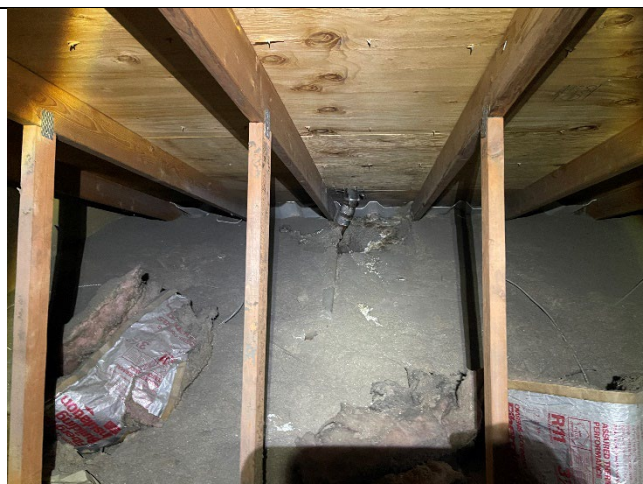
Aurora Harbor Office: View of misc broken bathroom vent through the roof at the main entry bathrooms. Vent is venting into attic space.
