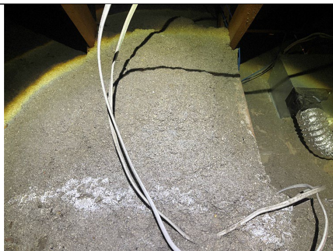
Aurora Harbor Office: misc loose wires common throughout attic space.
