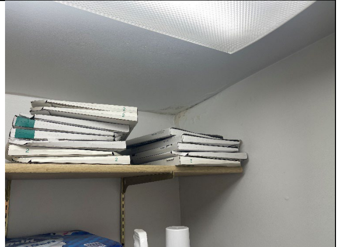
Aurora Harbor Office: South bathroom water damage at ceiling and walls from broken vent pipe through the roof.
