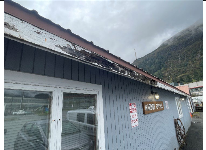
Aurora Harbor Office: General view of East side exterior water damage. Excessive wood decay present.
