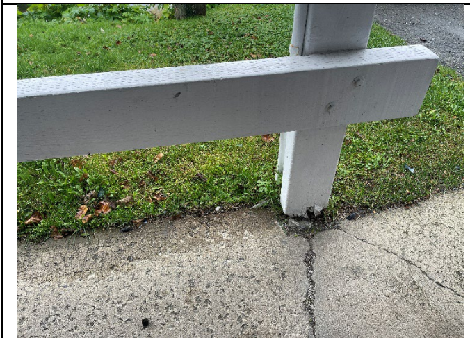
Aurora Harbor Office: Base of existing exterior canopy columns show signs of water damaged and are deteriorating.
