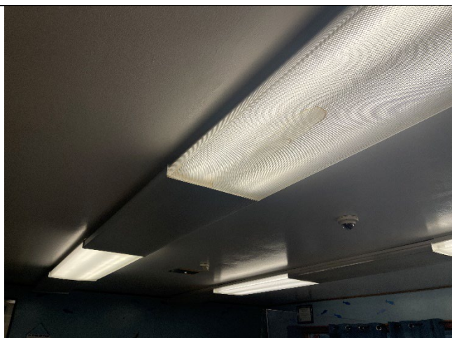
Aurora Harbor Office: Signs of water intrusion in light fixtures above the main office area.
