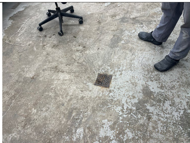
Aurora Harbor Office: Typical floor drains in the office (old garage area) smell of sewer gases.
