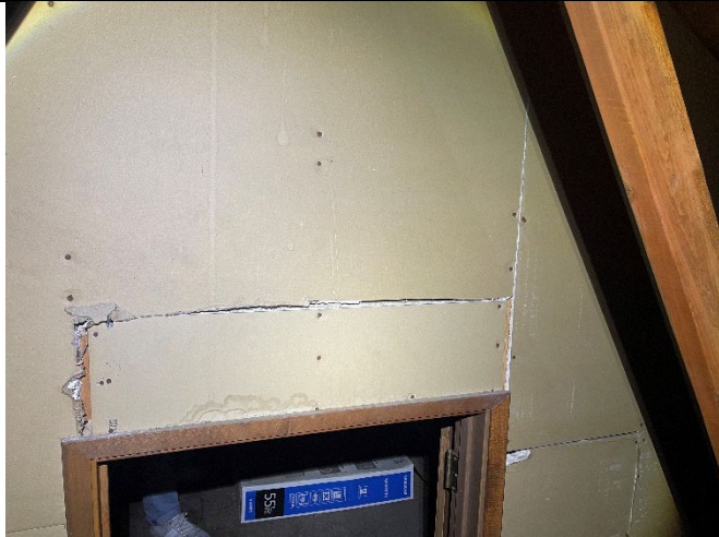
Aurora Harbor Office: Gypsum and any joint compound present should be tested for presence of ACM both attic and office areas.
