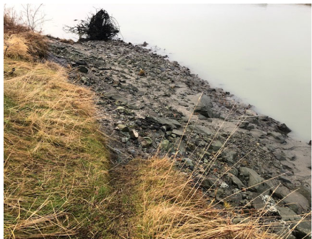
Photo 02: Damaged area looking down river. Rock loss ends near the tree root ball shown at top of photo.
