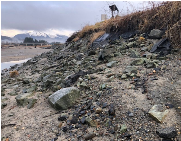
Photo 01: Damaged area looking to the north (upriver). Rock loss begins below the signs shown at upper right.
