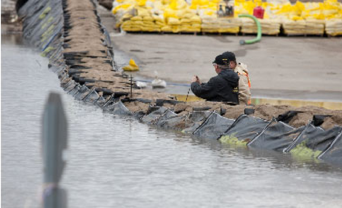
Sand filled Levee System
