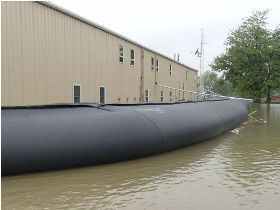
Water Filled Sandbag Equivalent Levee
