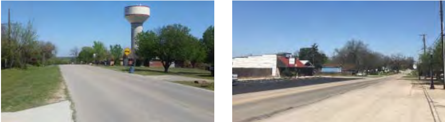
Figure 9: Existing Site Photos Show Lack of Sidewalks
