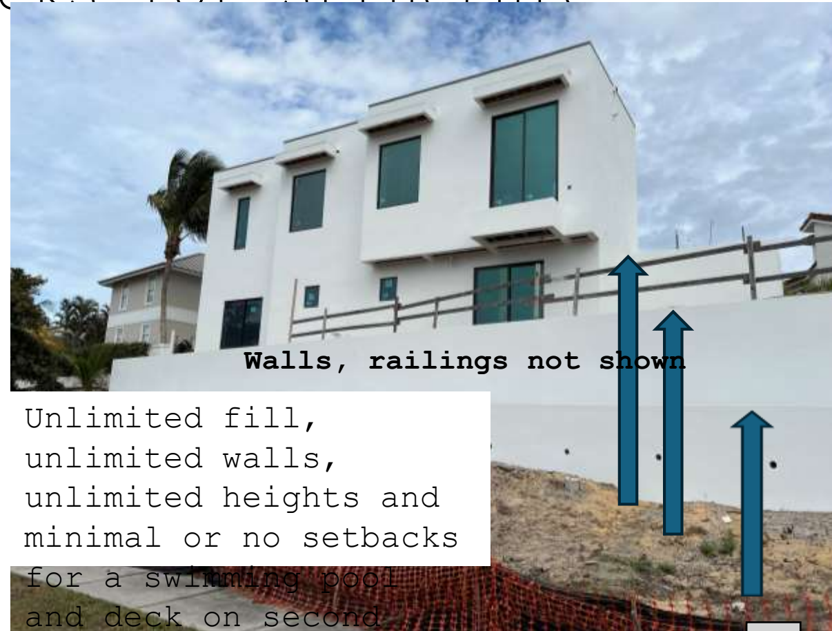
Series of Walls: front and side yard total of 15 feet in height in the side yard (11 ft wall with 4' railing) without meeting setback requirements for
