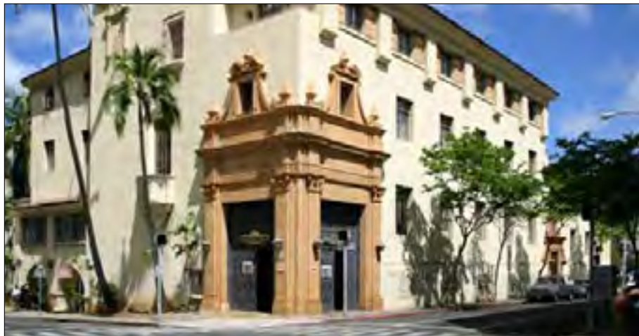
Figure 39 Old Police Station, Honolulu, Hi.
