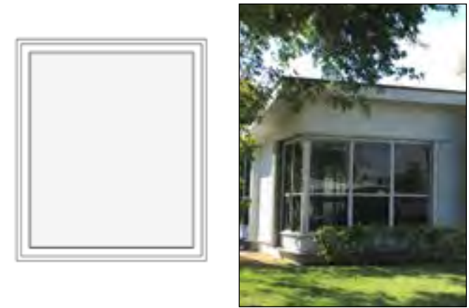
GROUPED FIXED-PANE WINDOWS WRAPPING A CORNER WITH A PIPE COLUMN
