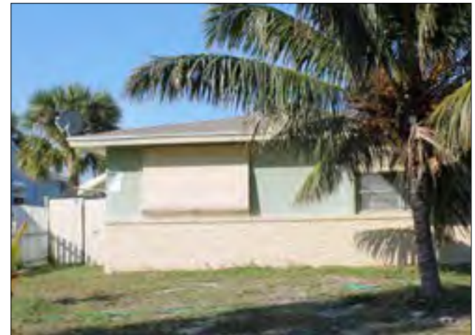
SMOOTH STUCCO WITH A CONTINUOUS BRICK BASE
