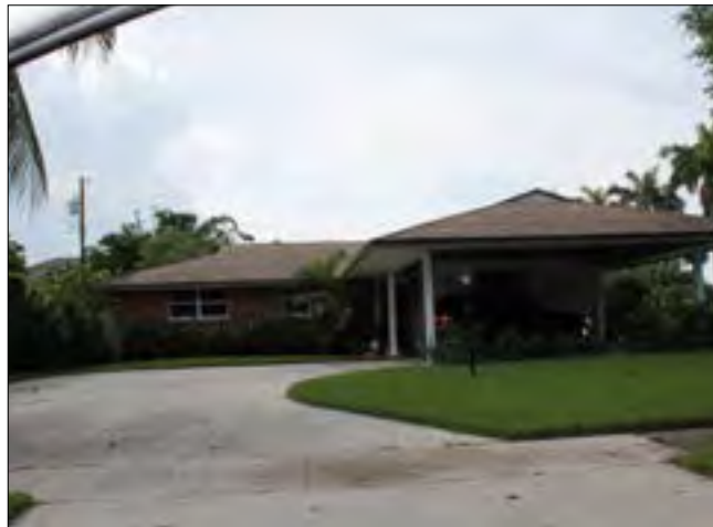
THIS RANCH HOME HAS ASPHALT SHINGLES & A DEEP PORTE-COCHERE
