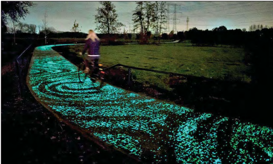
Starry Night Bike Path in the Netherlands uses glow-in-the-dark technology and solar-powered LED lights to light the way on this 600-meter trail in Eindhoven. © 2014 Daan Roosegaarde. Image Source: http://www.solaripedia.com/13/413/starry_night_solar_bike_path_(netherlands).html
