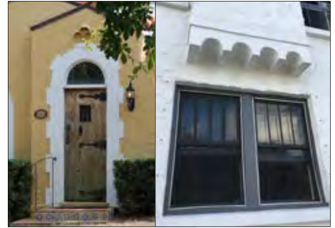
DECORATIVE STUCCO DETAILS AROUND WINDOWS & DOORS
