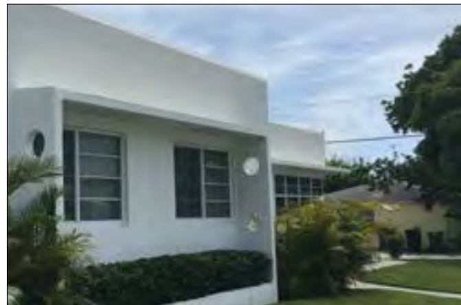
PORTHOLE OPENINGS IN DECORATIVE WING WALLS
