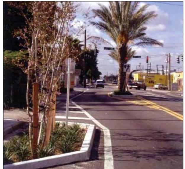
Bulb-out and median create a lateral shift in the travel route. Image courtesy of Ian Lockwood.
