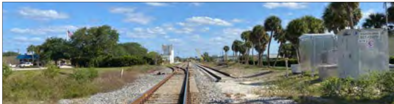
FEC Railway view South near the intersection of Tequesta Drive.
