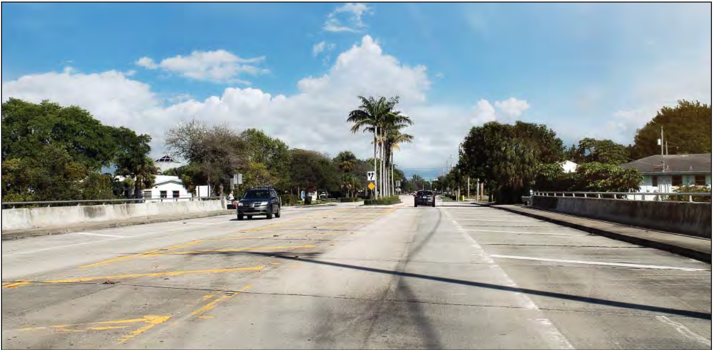
A view of the current bridge on Prosperity Farms Road over the Earman River.
