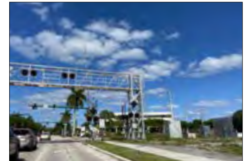
View of the FEC railway crossing at Tequesta Drive (looking West).
