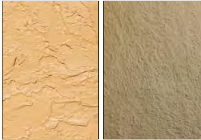
STUCCO TREATMENTS ARE TYPICALLY MEDIUM TO ROUGH IN TEXTURE
