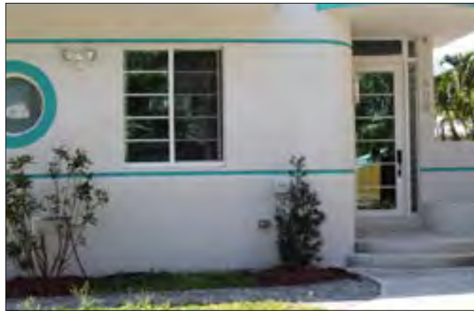
LARGE PORTHOLE WINDOW & CANTILEVERED EYEBROWS OVER THE WINDOWS AND ENTRY
