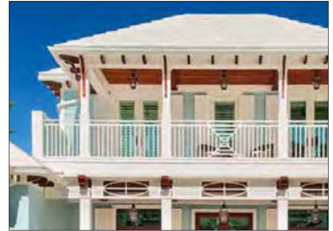
EXPOSED RAFTER TAILS AND BRACKETS WITH DECORATIVE WOODEN RAILINGS AND CARVED WOOD DETAILS
