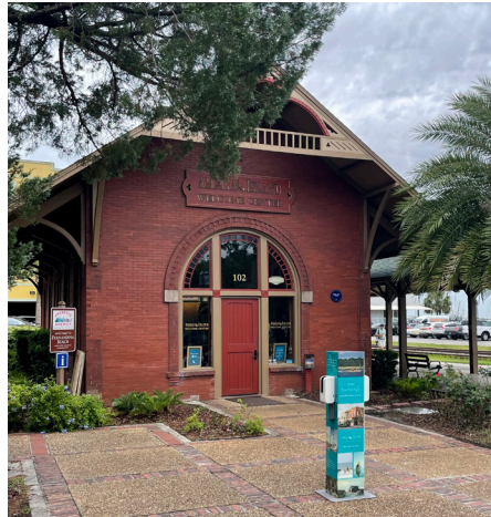
Photo: Historic Structures in Fernandina Beach (Source: WGI)
