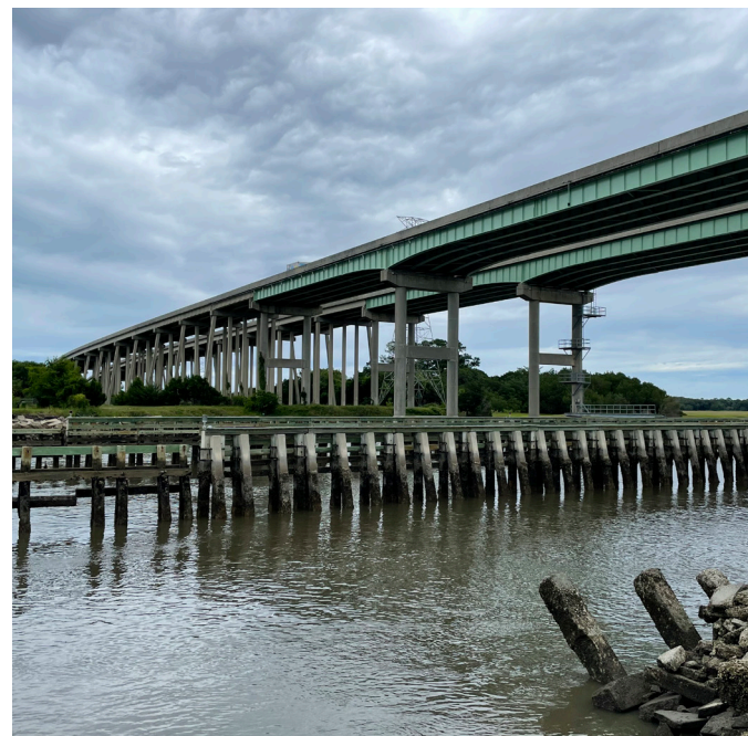
Photo: Thomas J. Shave Jr. Bridge (source: WGI)
