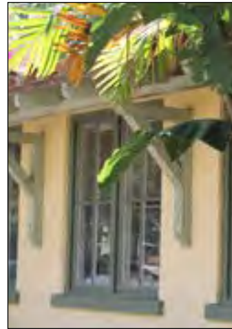
MULTI-LIGHT WOODEN CASEMENT WINDOWS
