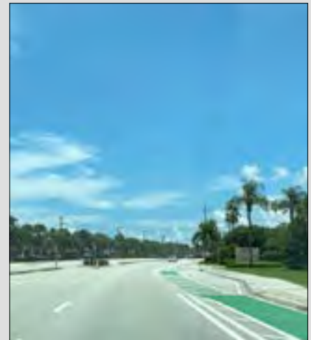
Existing conditions along US-1
