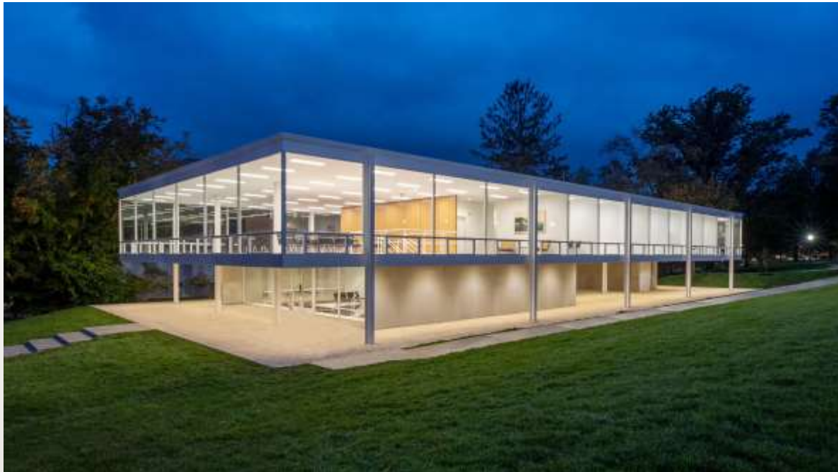
ESKENAZI SCHOOL OF ART, ARCHITECTURE DESIGN, INDIANA UNIVERSITY SIMPLE COLOR PALLET, LIGHT MATERIALS, SIGHT LINES USING CEILING TO FLOOR GLASS SLEEK VERTICAL LINES, SINGLE HORIZONTAL PLANE CREATION OF NEGATIVE SPACE ON FIRST FLOOR GEOMETRIC SHAPES
