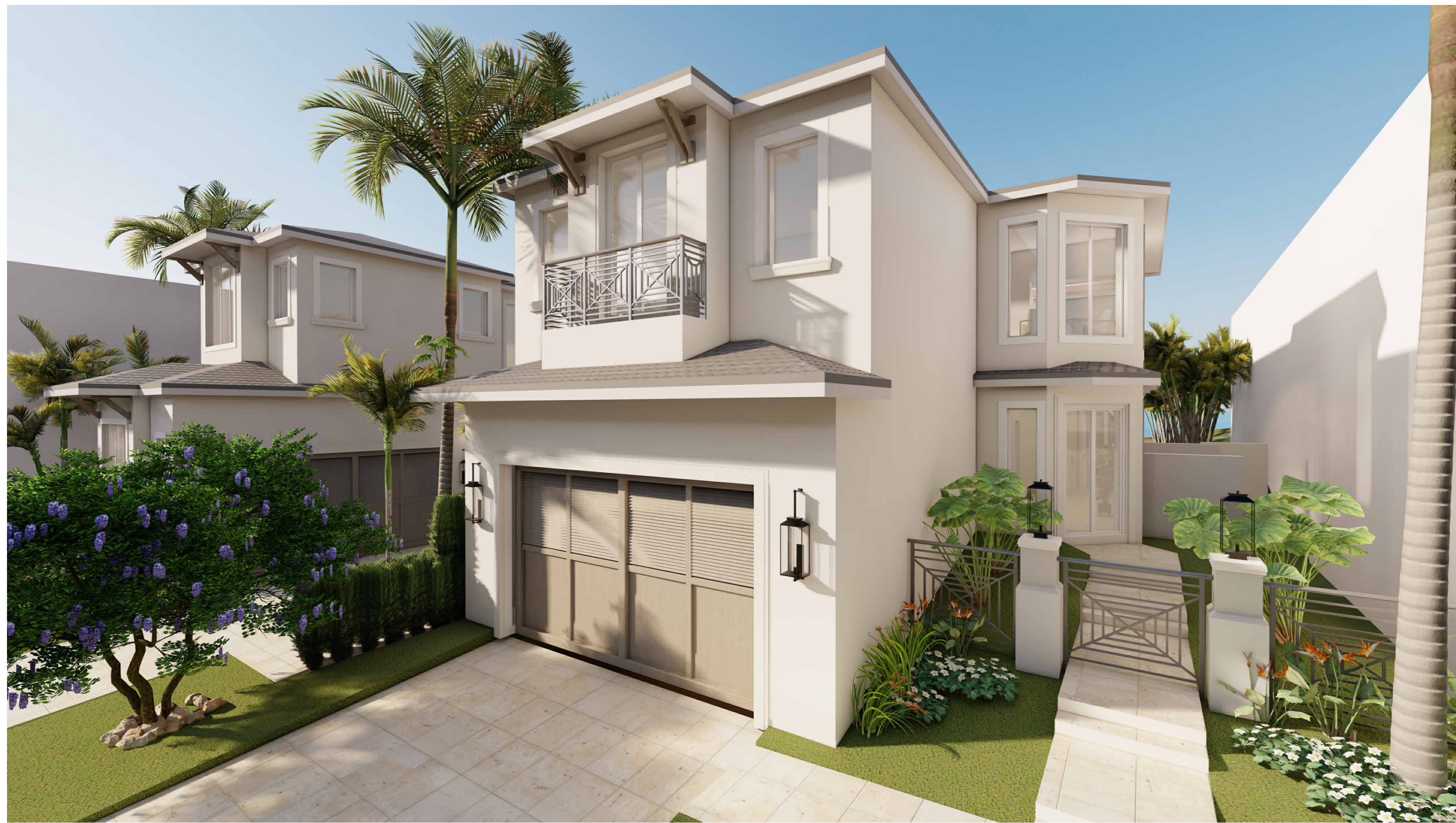
PROPOSED 714 ENTRY **REFER TO LANDSCAPE ARCHITECTURAL PLANS FOR LANDSCAPE AND HARDSCAPE DESIGN
