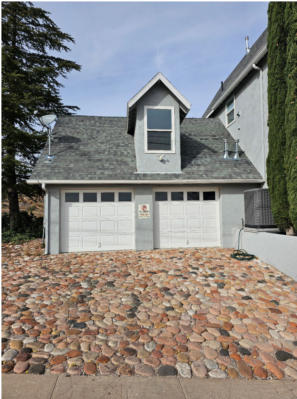
Top: View of 778 East avenue from the street looking west, close up on the attached garage. Note the Shed Dormer which sits off-center from the garage.
