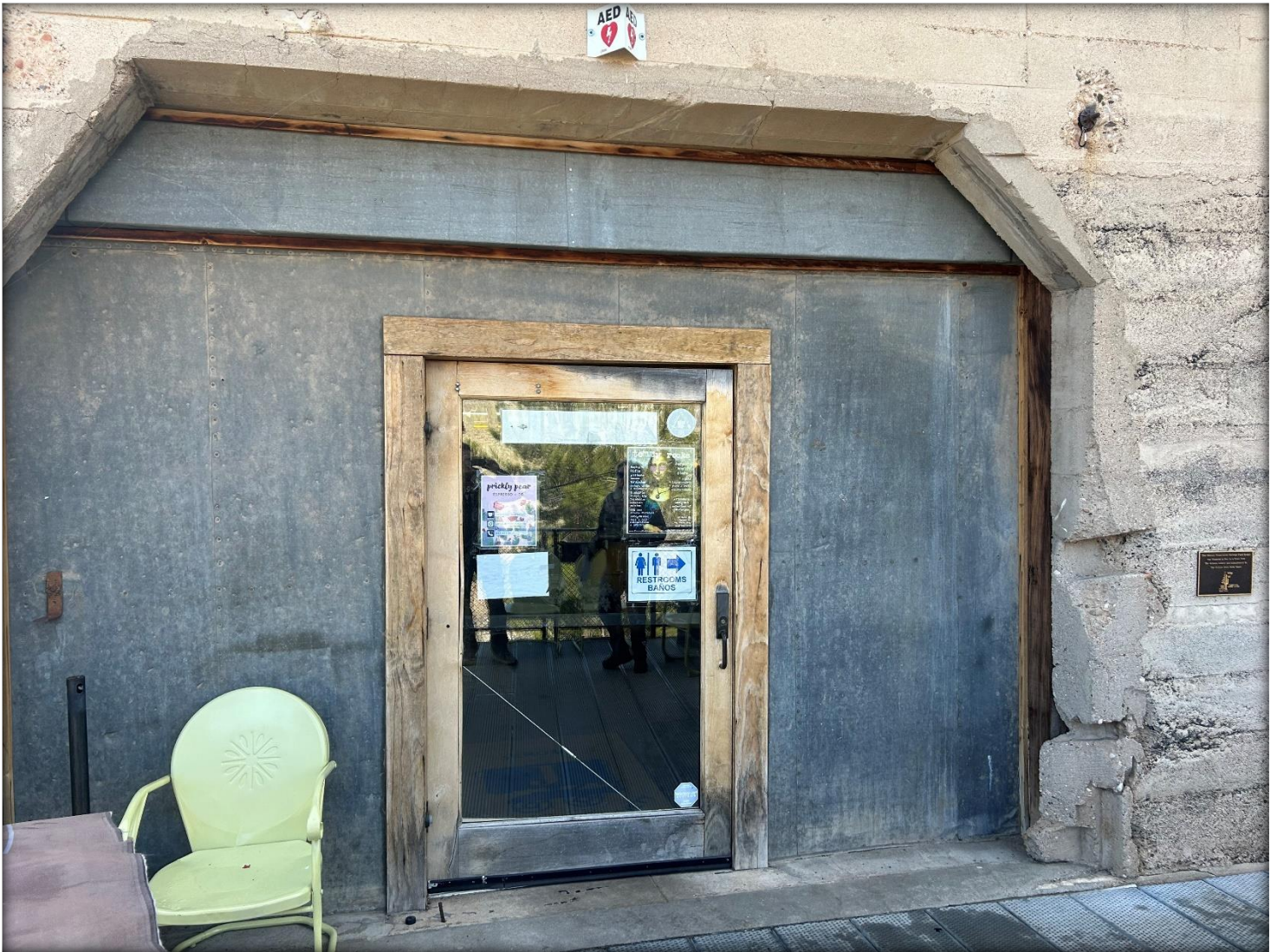
View of the existing door leading into the mid-level of the New State Motor Building shops.
