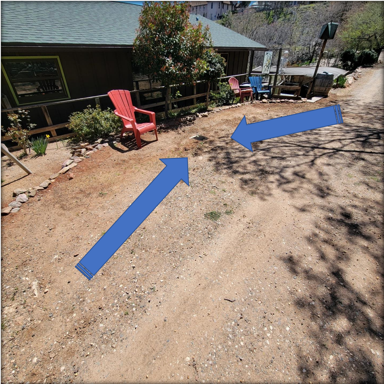
View showing the direction of water flow / drainage that has been negatively impacting the residence. The drainage patter will be addressed by the Town crew. Source: W. Blodgett
