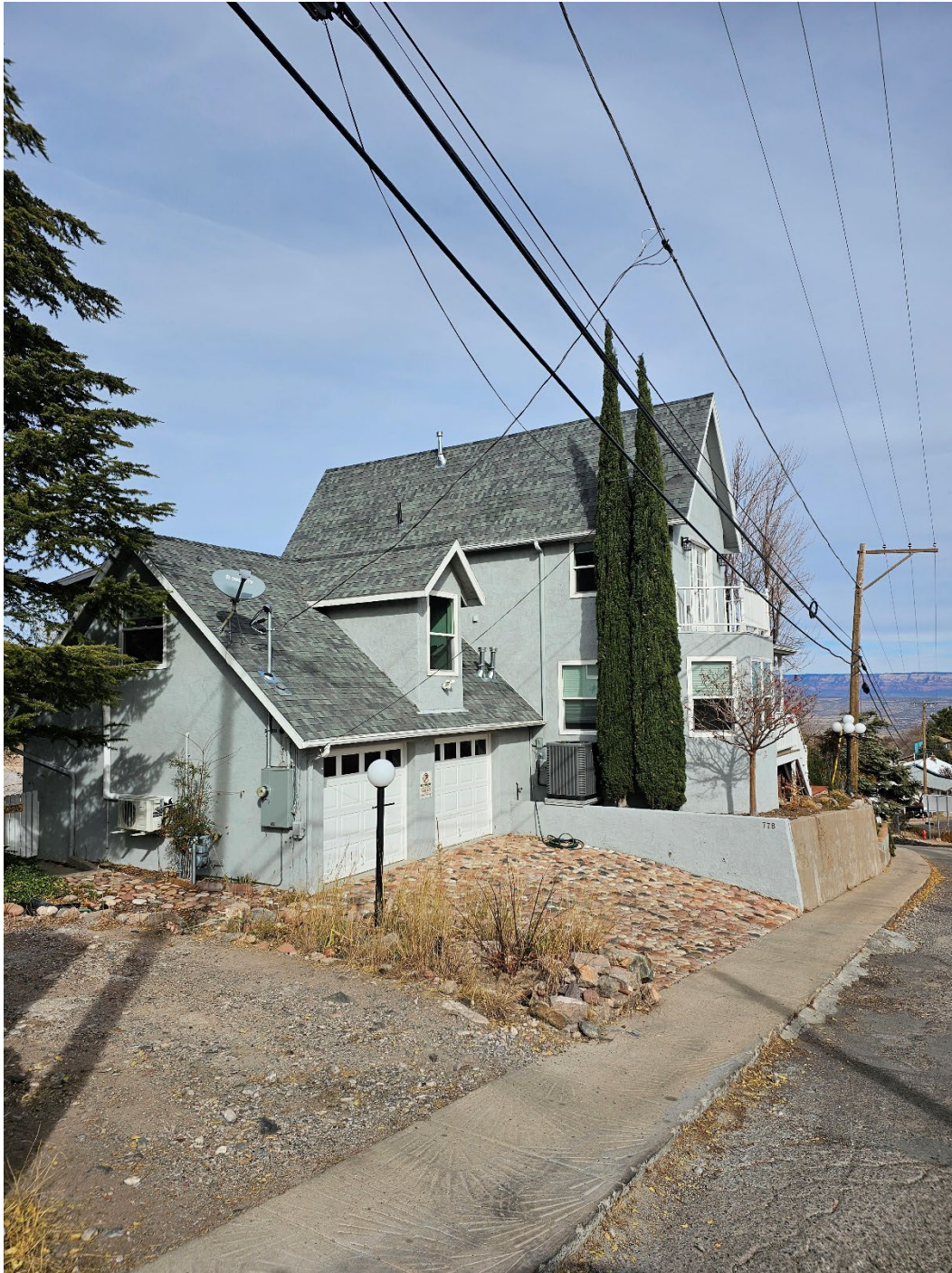
Top: View of 778 East avenue from the street looking north. Note the attached garage which marks this as a modern construction.
