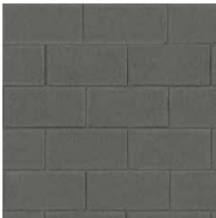
PAINTED SMOOTH-FACE CMU
