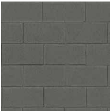
PAINTED SMOOTH-FACE CMU
