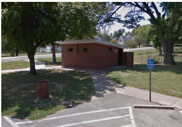
Figure 1: Existing Restroom (to be replaced)
