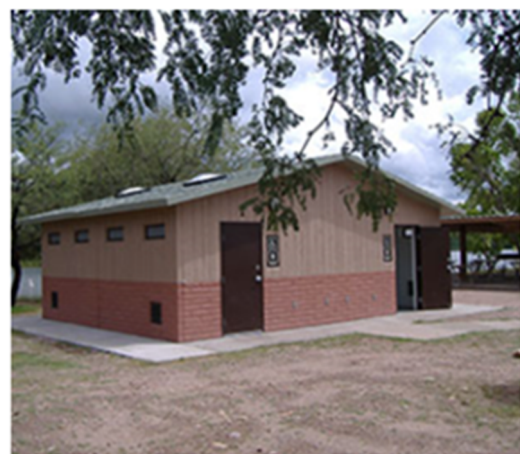
Figure 2: New Restroom Example
