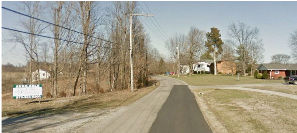
Figure 4: Northbound Curvature Approach
