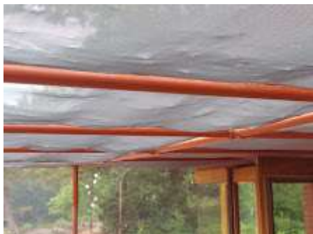
CR hail damage 2023 RP copper screen.jpg 5601K
