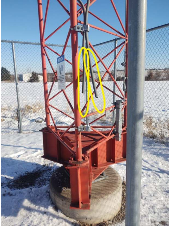
Tower Ground Bar after Repair
