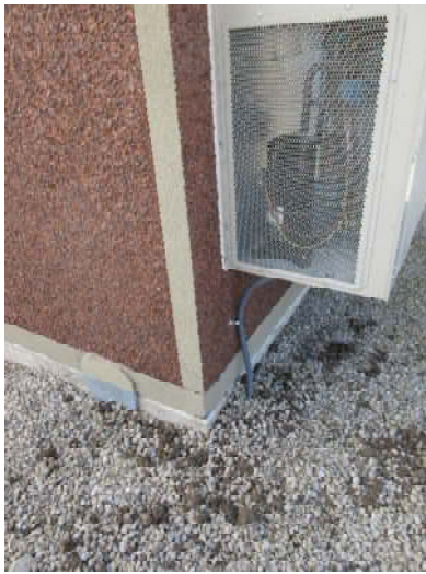
HVAC Ground after Repair
