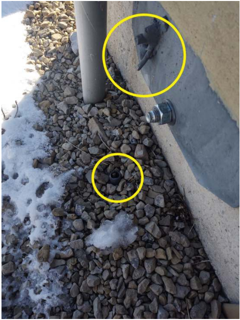
Shelter SE Corner Ground Missing
