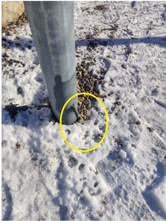
Ice Bridge Post #6 Ground Missing
