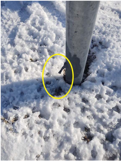
Ice Bridge Post #4 Ground Missing
