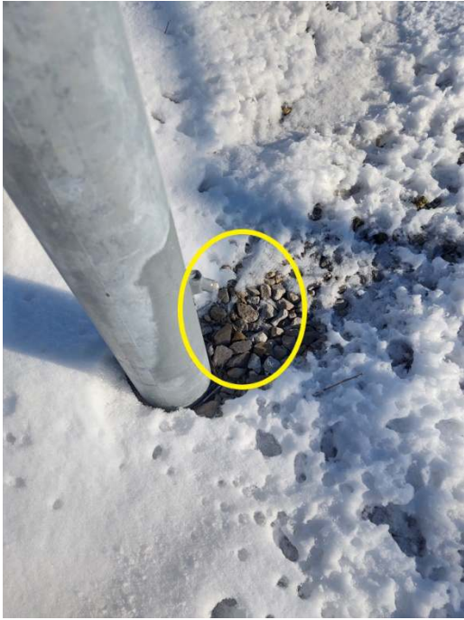
Ice Bridge Post #4 Ground Missing
