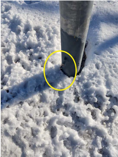
Ice Bridge Post #2 Ground Missing
