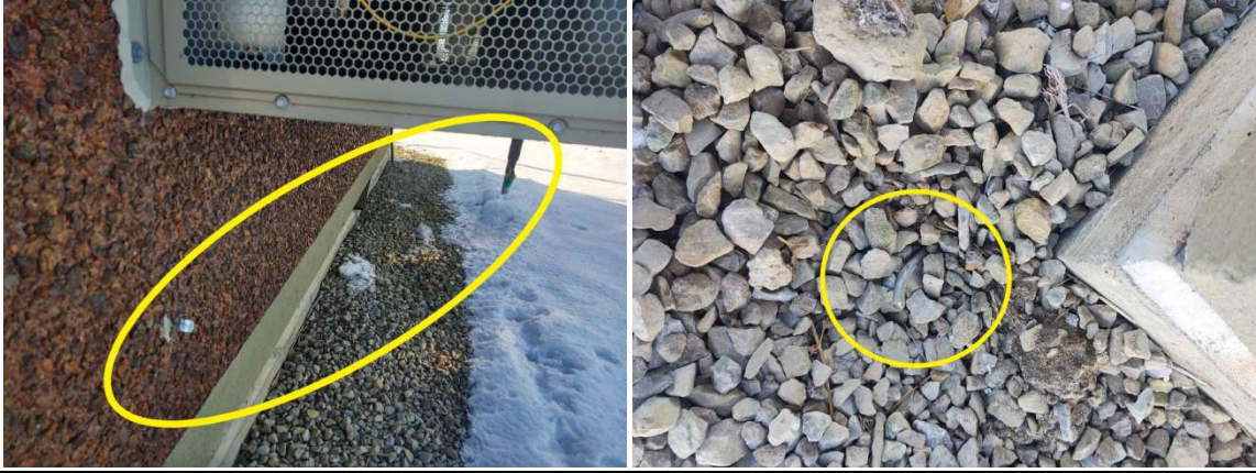
Shelter SE Corner Ground Missing
