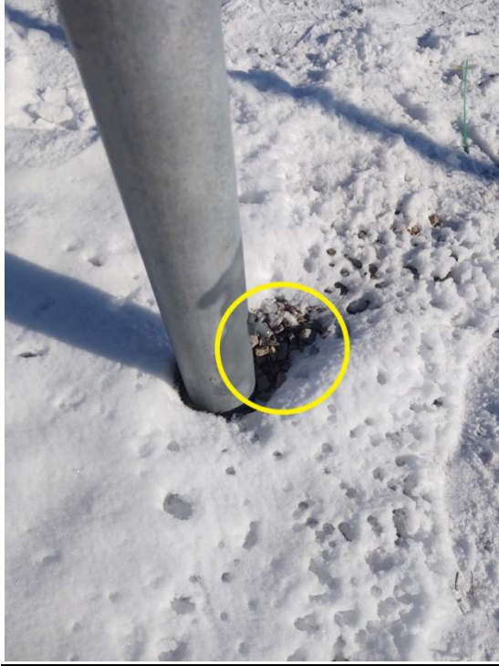
Ice Bridge Post #6 Ground Missing
