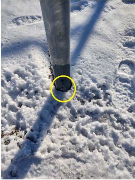
Ice Bridge Post #2 Ground Missing
