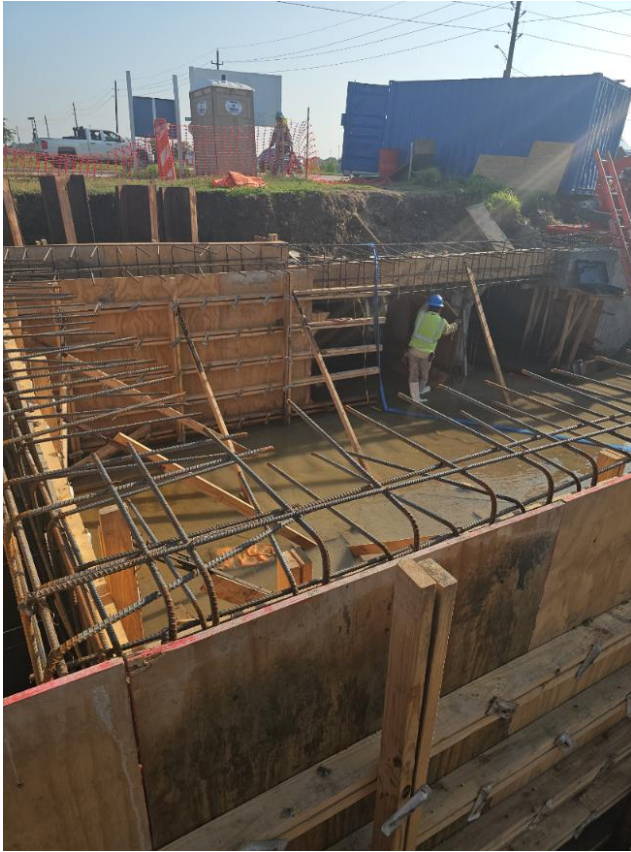
Figure 1: Rebar Inspection for junction box wall
