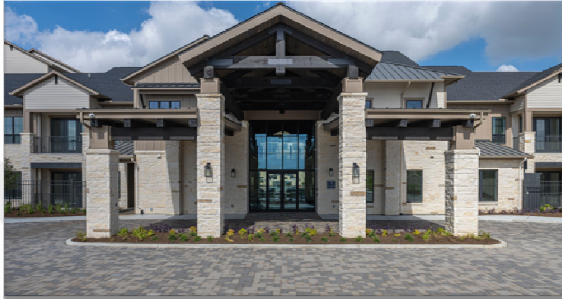
Representative photo of standard Cadence multistory building
