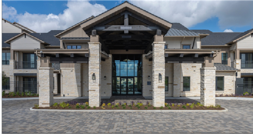
Representative photo of standard Cadence multistory building
