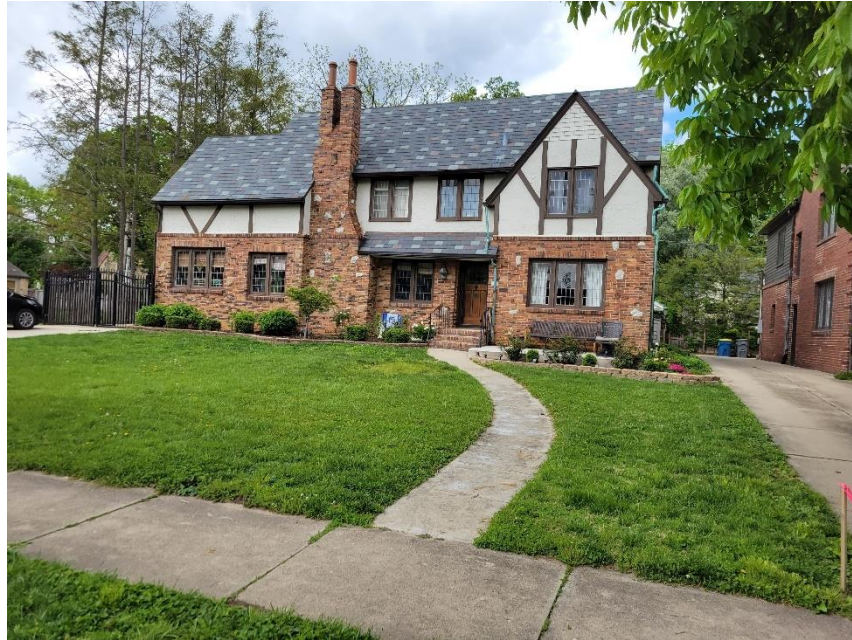
Photo 1: Subject Property Viewed from South
