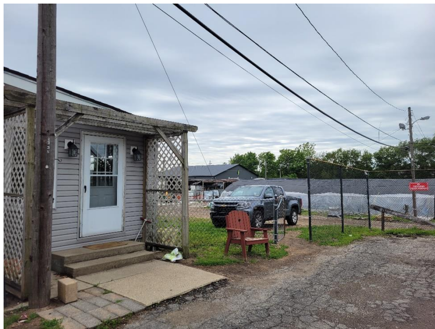
Photo 10: Contractor Use (2401 Morris) Viewed from Northeast (Alley)
