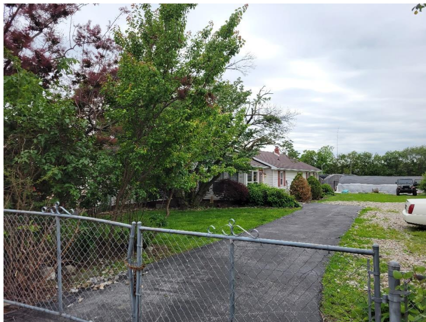
Photo 6: 1220 Tremont Viewed from Northeast
