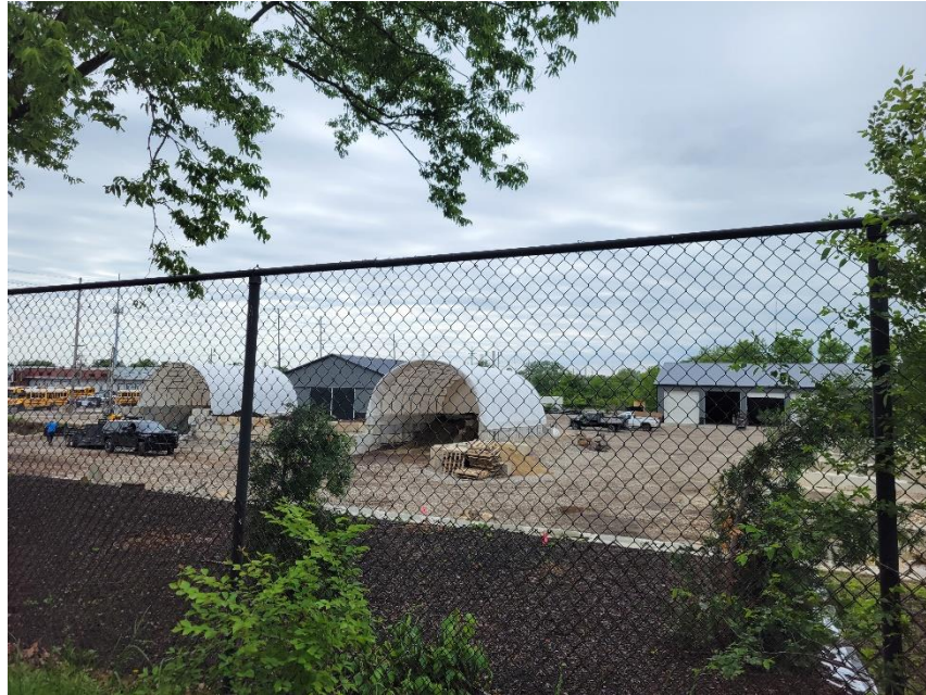
Photo 11: Contractor Use (2401 Morris) Viewed from East
