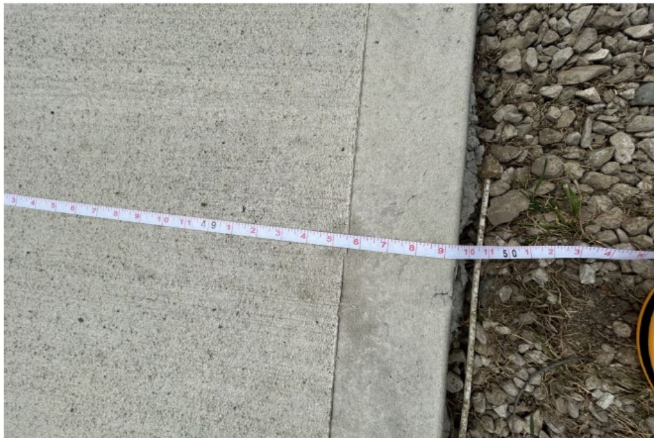
Photo 1: Inspector photographs showing the width of the driveway beyond 30 feet
