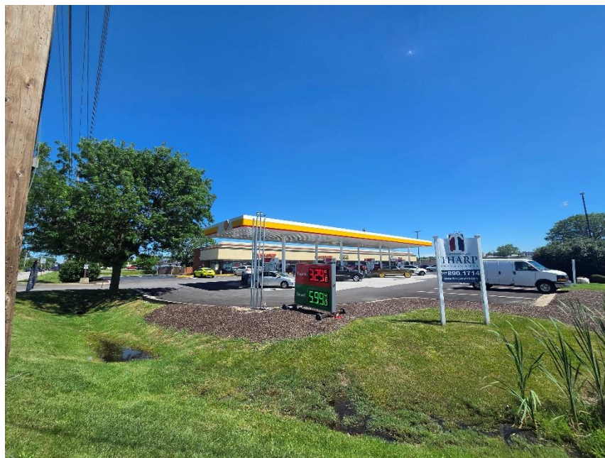
Photo 2: Extended Canopy Viewed from Northwest
