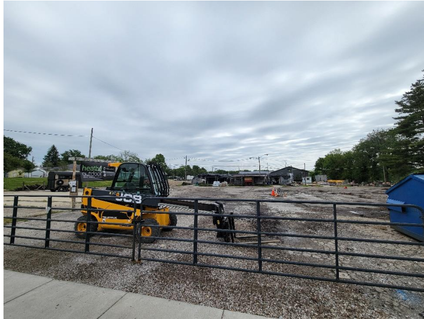
Photo 9: Contractor Use (2401 Morris) Viewed from North
