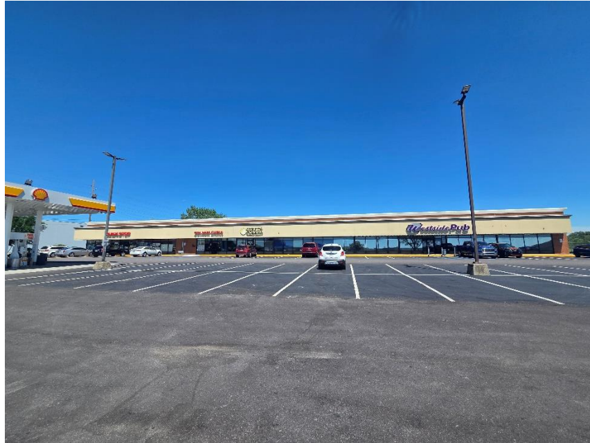
Photo 3: Existing Multitenant Commercial Building Viewed from West
