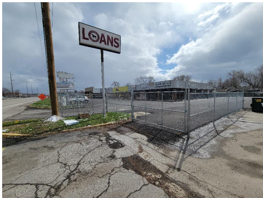
Photo 2: Subject Fence Viewed from Northwest
