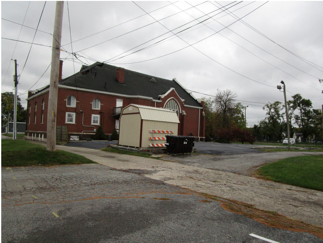
View from site looking southeast at intersection of the alleys abutting the site to the east and south
