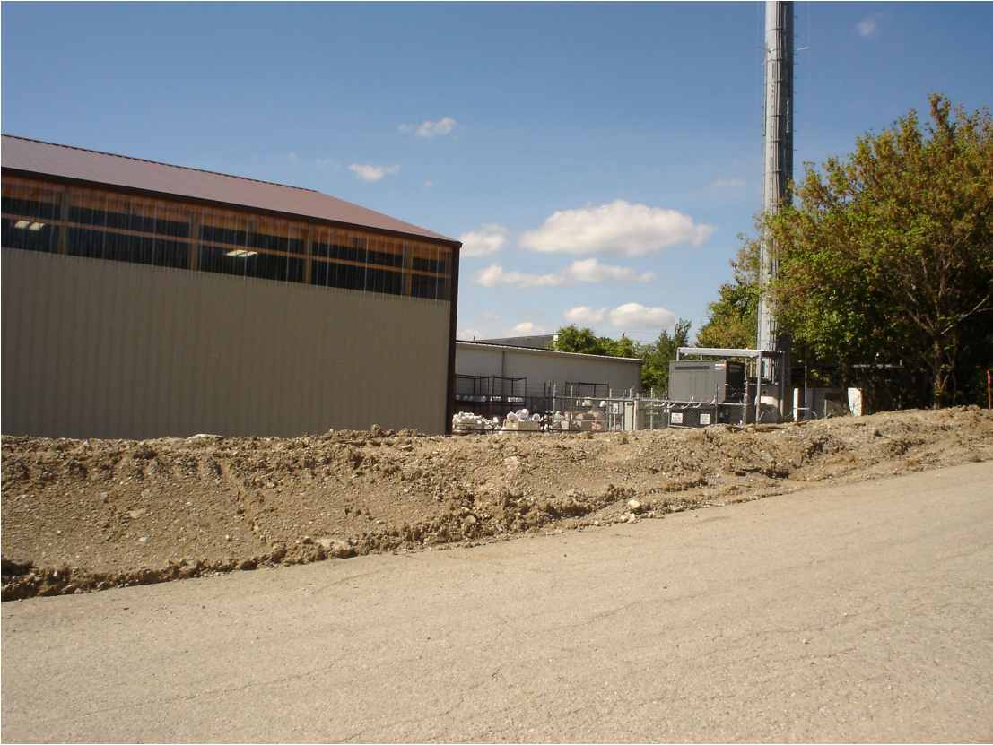
View from site looking northwest at adjacent property.
