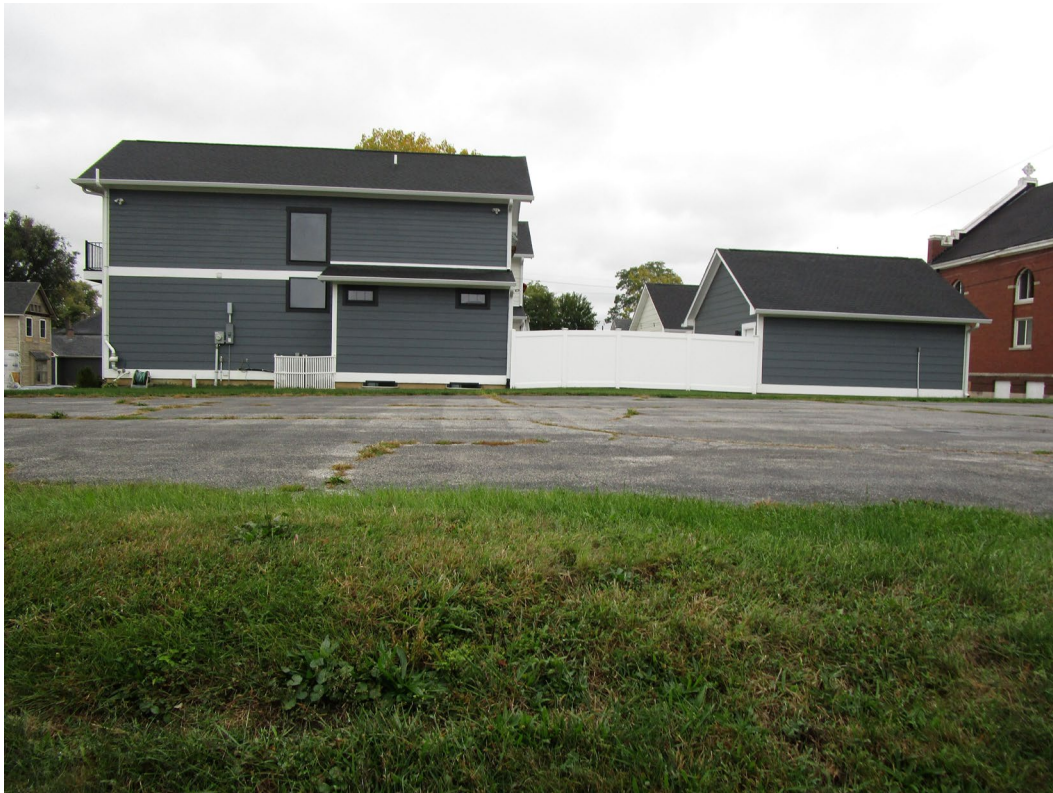
View of parking lot (addressed as 217 Orange Street) looking south
