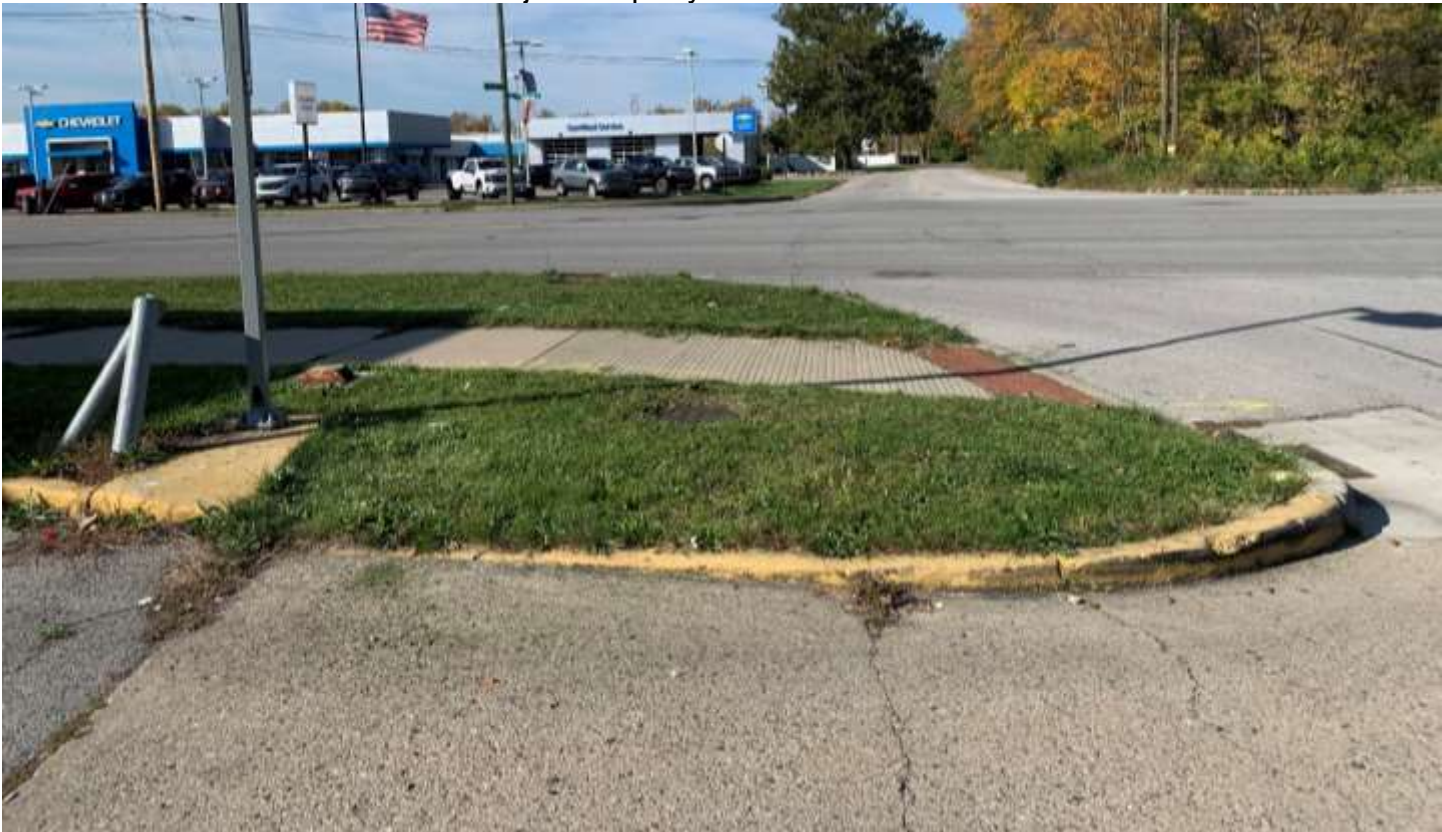
Location where a pedestrian safety island and pedestrian-activated crossing signal was proposed.
